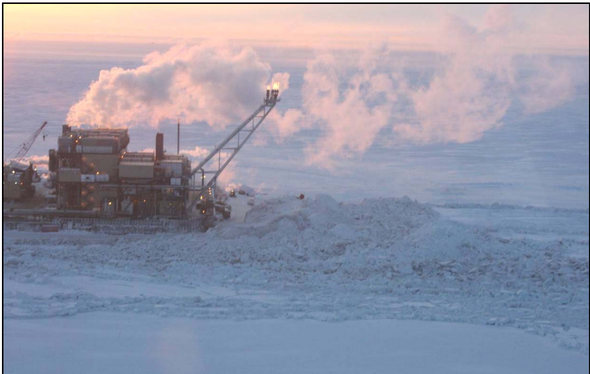
Plate 1. Ice Pile-Up Formed on Northstar Production Island in January, 2008 (Coastal Frontiers, 2009)
