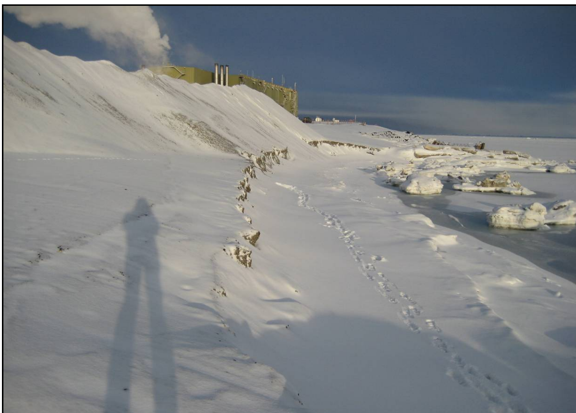
Plate 7. Ice Cover on East Side of Prudhoe Bay West Dock, October 20, 2011
