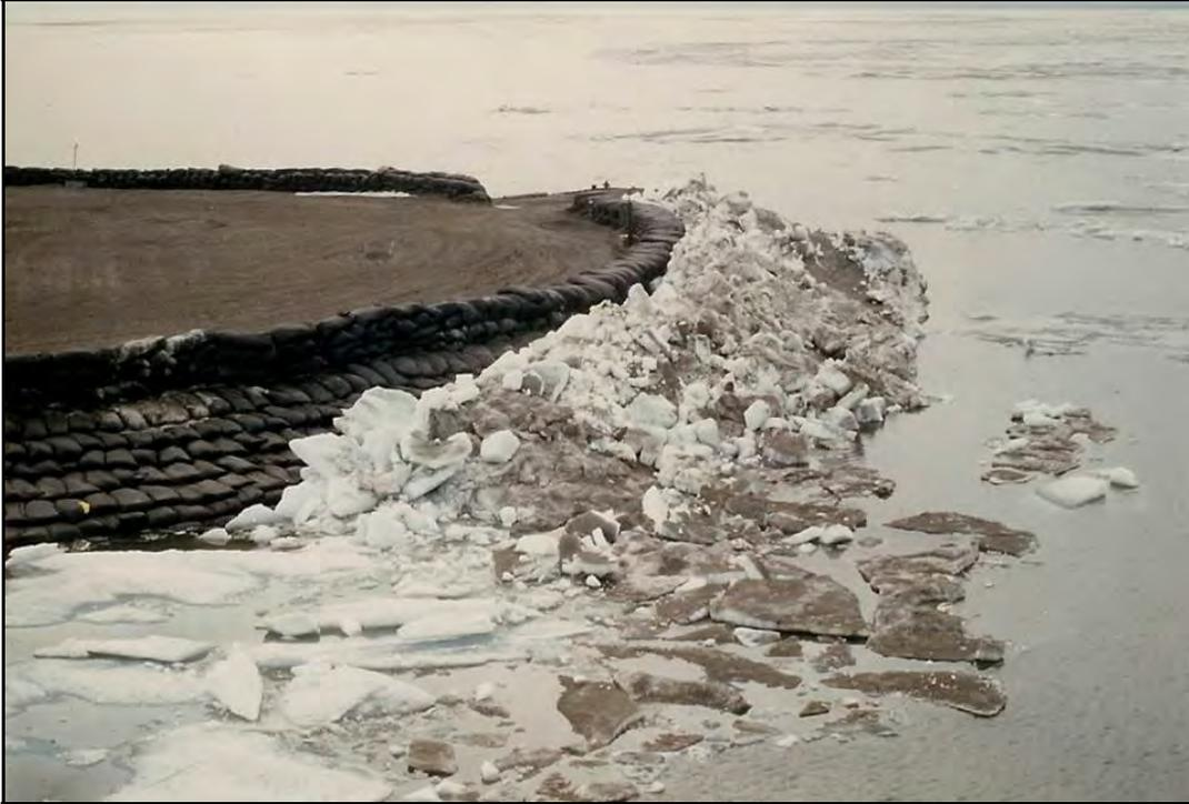
**Plate 17. 6.9-m Pile-Up on Tern Island in Early July 1984 (60-120 cm thick ice blocks encroached 14 m onto gravel bag armor during 20- to 25-kt westerly storm.)**
