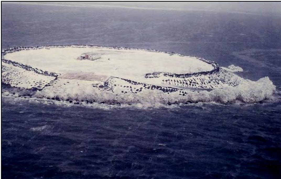
**Plate 11. 6.1-m High Ice Pile-Up on Seal Island that Resulted from SW Storm on October 19, 1982.**
