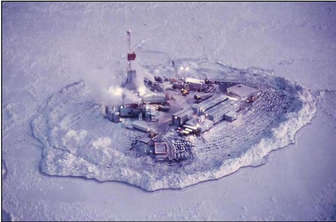
**Plate 19. 7.6-m Pile-Up on Mukluk Island in Late November 1983 (60-65 cm thick ice blocks piled up at waterline during 30- to 35-kt easterly storm.)**
