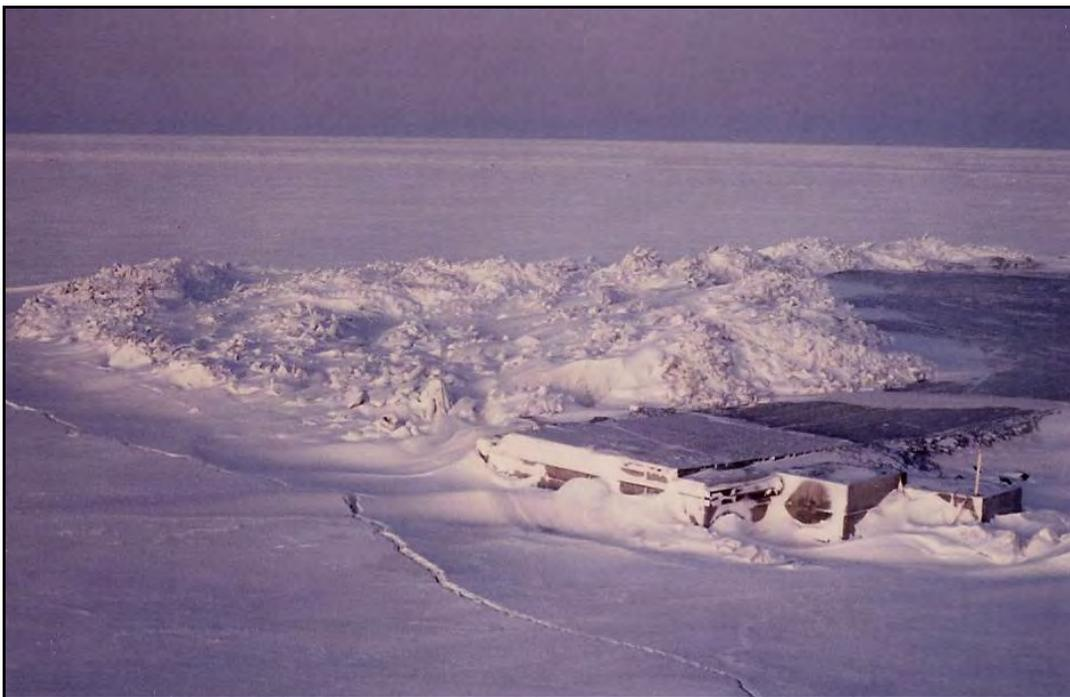
**Plate 9. 7.6-m High Ice Pile-Up on Endeavor Island in Mid-October 1982 (20-cm blocks encroached 5 m onto work surface during 40-kt SW storm.)**
