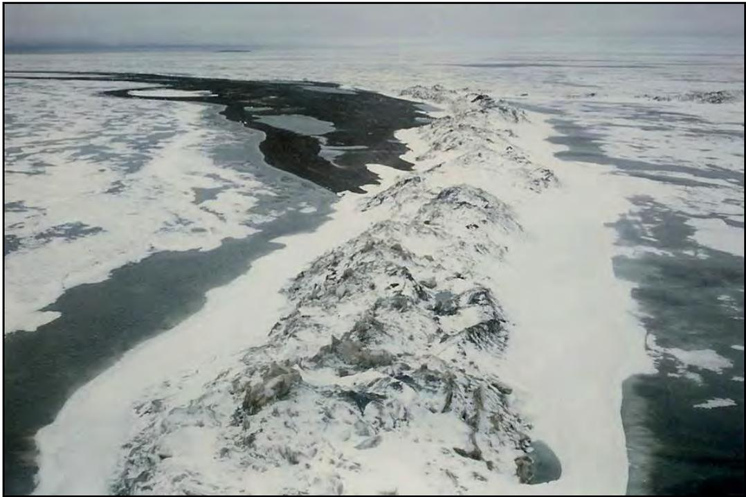
**Plate 26. 10.6-m Pile-Up on Spy Island in Early December 1982 (60-90 cm thick ice blocks encroached 36 m across full width of island during 20- to 25-kt easterly storm.)**
