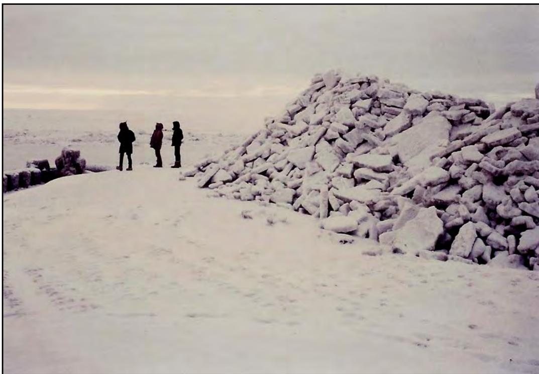
**Plate 16. Work Surface Encroachment of 6 m on Tern Island in Mid-October 1984**
