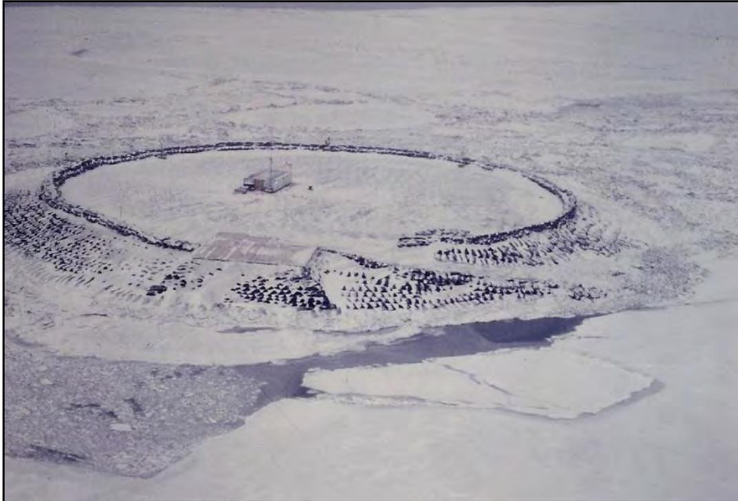
**Plate 10. Broken Ice and Open Water around Seal Island on October 18, 1982 after Easterly Storm**
