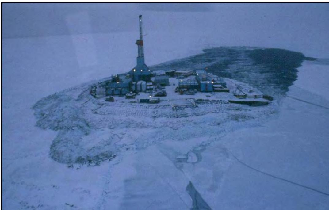
**Plate 20. 11.5-m Pile-Up on Sandpiper Island in Mid-November 1985 (50-cm thick ice blocks encroached 5 m onto gravel bag armor during 30- to 40-kt westerly storm.)**
