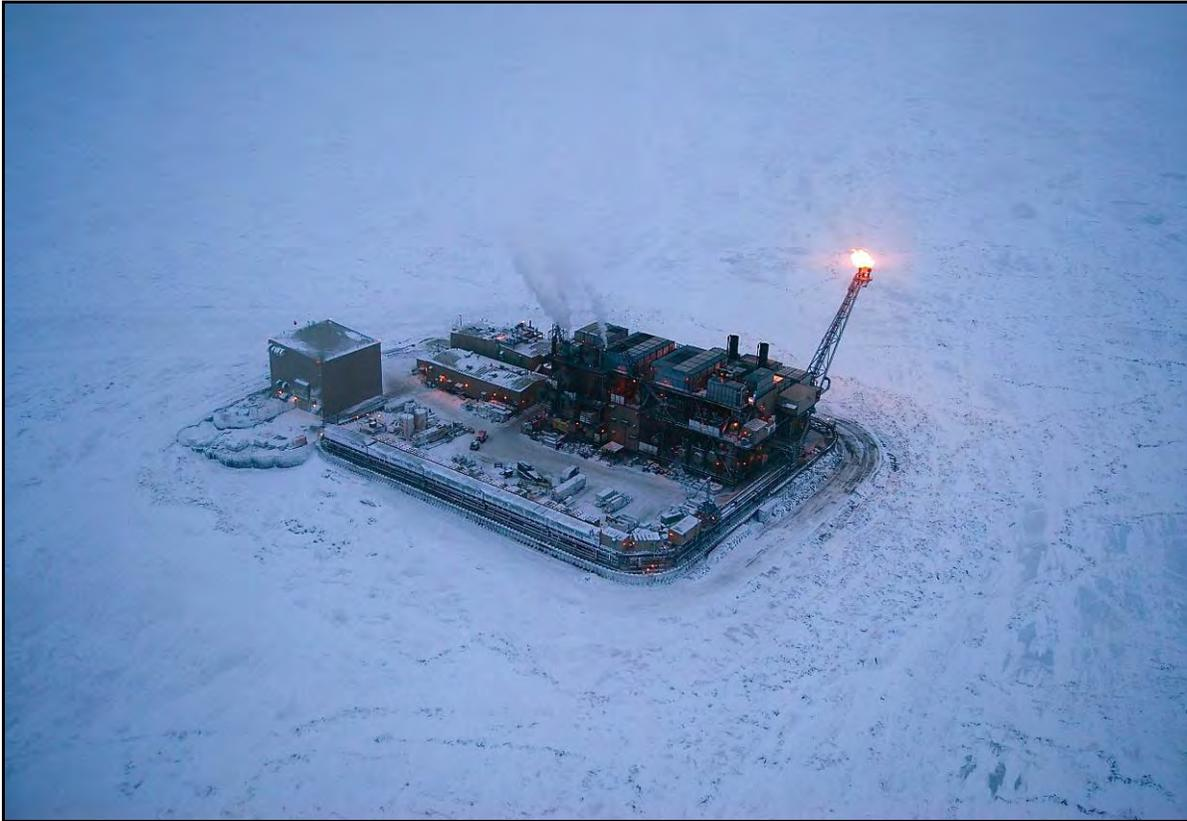
**Plate 29. 4-m Pile-Up on Northstar Production Island in mid-November 2011 (30-cm thick ice blocks encroached 5 m onto concrete mat during 15- to 25-kt westerly storm)**
