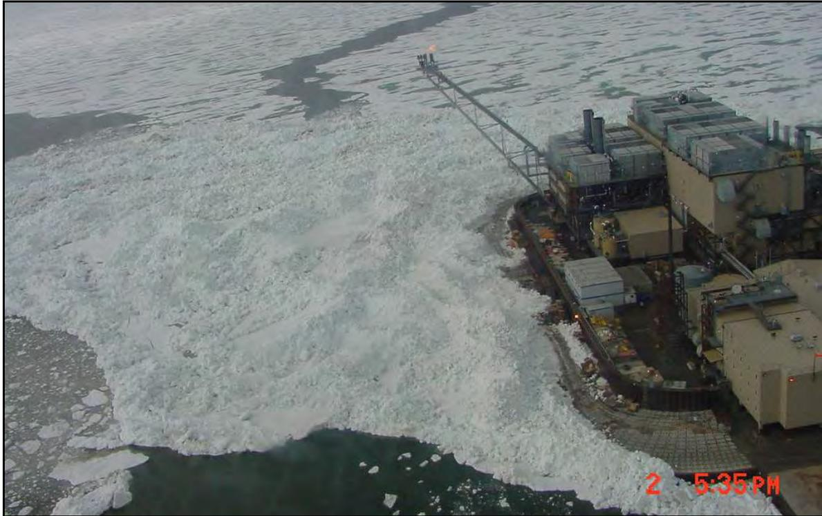
**Plate 22. 9.1-m Pile-Up on Northstar Prod. Is. in Early July 2002 (1.0-1.5 m thick ice blocks encroached 27 m onto concrete mat during 10- to 20-kt westerly wind.)**
