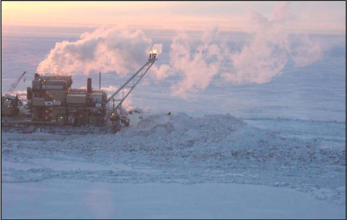
**Plate 21. 14.3-m Pile-Up on Northstar Production Island in Late January 2008 (60-90 cm thick ice blocks encroached 27 m onto concrete mat during 30- to 40-kt westerly storm; Coastal Frontiers, 2009.)**
