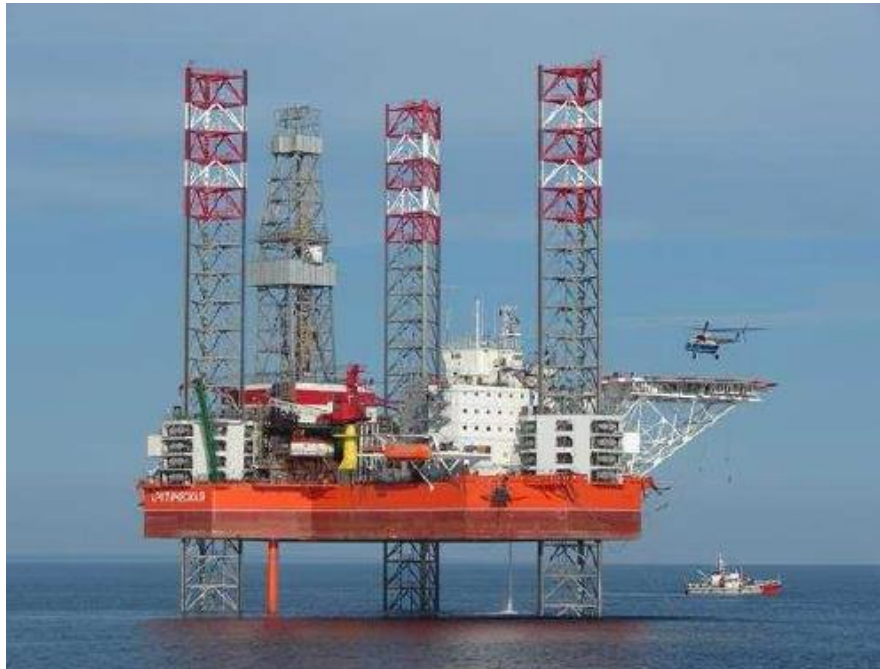
Figure 2.12: Jack-up Drilling Rig
