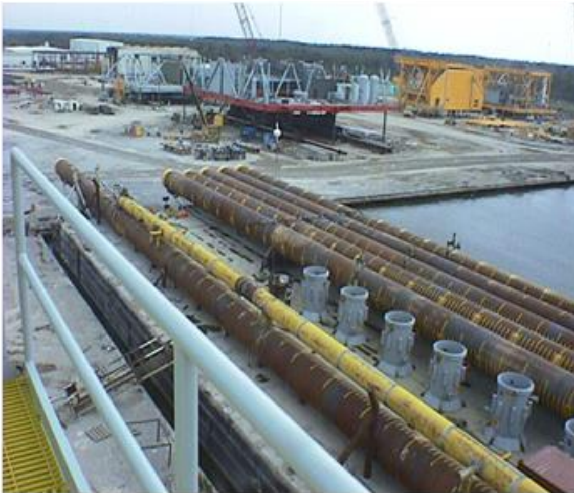
Figure 2.6 - Piles with receptacles attached. The CP anode sleeves shown are installed after pile driving. (Photo courtesy of ENI)
