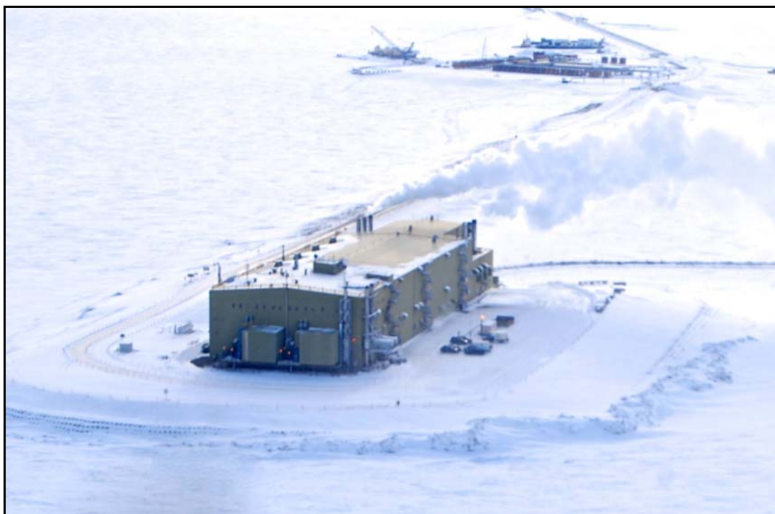
Plate 18. 8-m Pile-Up that Encroached 20 m onto Northwest Corner of STP Pad (looking south on March 30, 2014)
