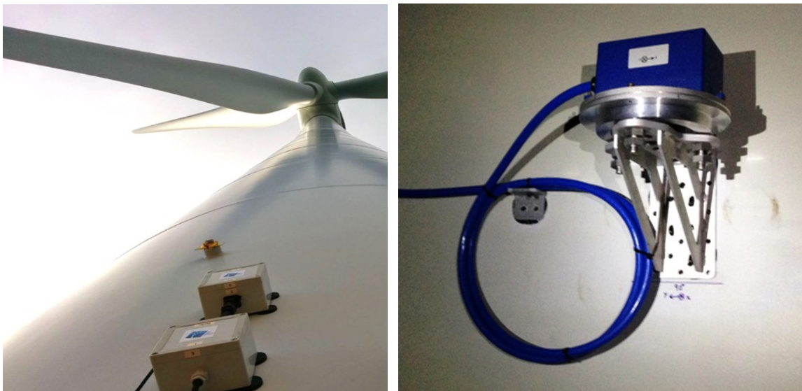
Figure 5-17 Left, accelerometers with magnetic footings (photo OWI-Lab) and mounting arrangement from NGI (combined accelerometer and inclinometer holder which can be turned)
