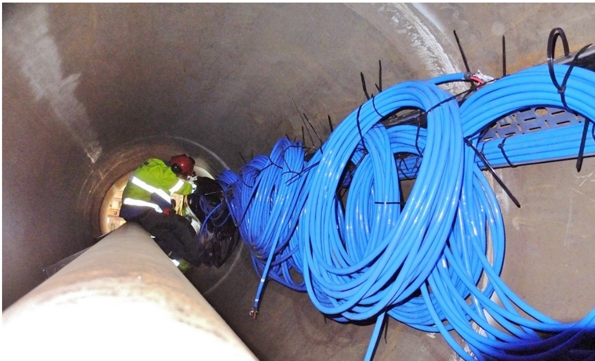
Figure 7-13 Long cables makes big bundles and even less work space before final routing (photo from NGI archives)
