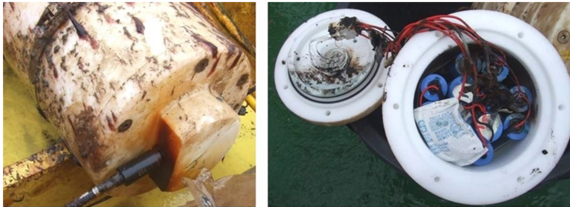
Figure 7-41 Burned batteries and galvanic corroded connector caused by stray currents in the water probably originating from broken cable isolation and fuses with insufficient sensitivity (Photo NGI archives)
