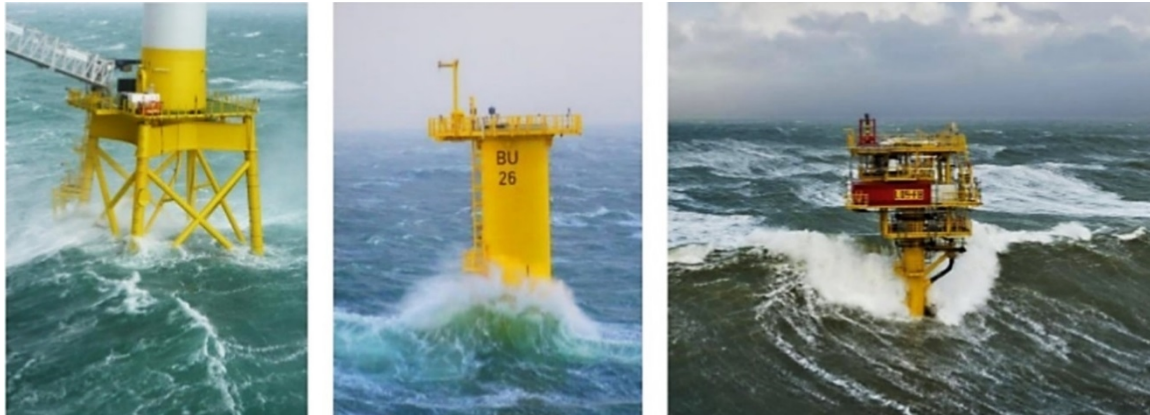
Figure 7-14 Battering wave action which can be expected in the splash zone (in the North Sea)
