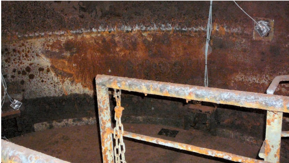
Figure 5-65 Corrosion is a severe problem for long term operation in the offshore environment, the photo shows the interior of a mono pile (courtesy Force Technology)
