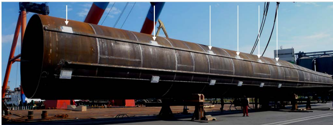
Figure 7-15 FINO 3 Mono pile with "GEMSOGS" instrumentation
