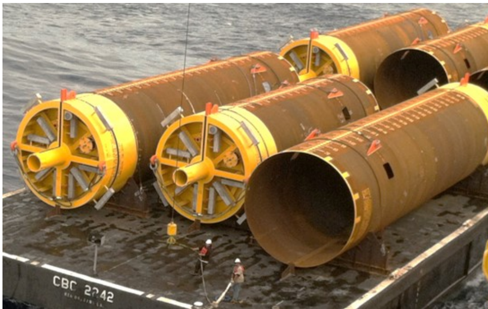
Figure 5-62 TLP suction anchors for a large floater
