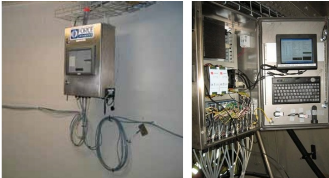
Figure 6-3 Example of compact wall mounted data acquisition cabinet inside TP serving small scale SHM systems (Force technology)
