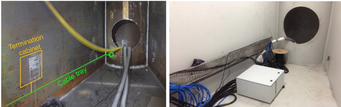
Figure 7-12 Example of cable routing details indicated during yard visit (left) and final installation (right), photo from NG's archives.
