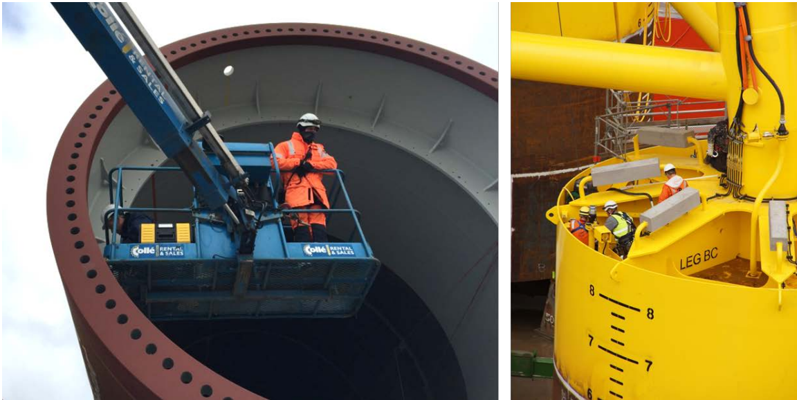
Figure 7-9 Access for installing sensors at the yard: Left, inside mono pile (photo: Allnamics) and right, on top of suction buckets (photo: NGI)
