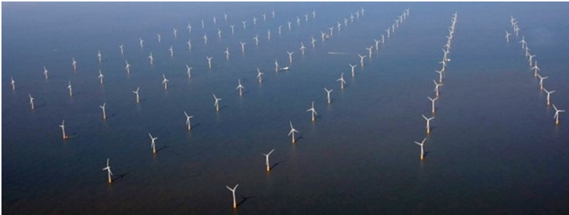
Figure 1-1 Presently the London Array wind farm located in the North Sea outside Kent is the largest in Europe with 175 OWT's producing 630 MW of power
