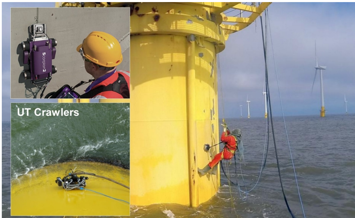
Figure 5-83 UT Crawlers for UT scanning (inserted pictures). The outside of for example the TP is not easily accessible, the large photo shows sand blasting at Scroby Sands wind farm with tie-back to the structure by a magnet system from Abfad. UT crawlers can be used for external UT scanning of TP's provided calm weather.
