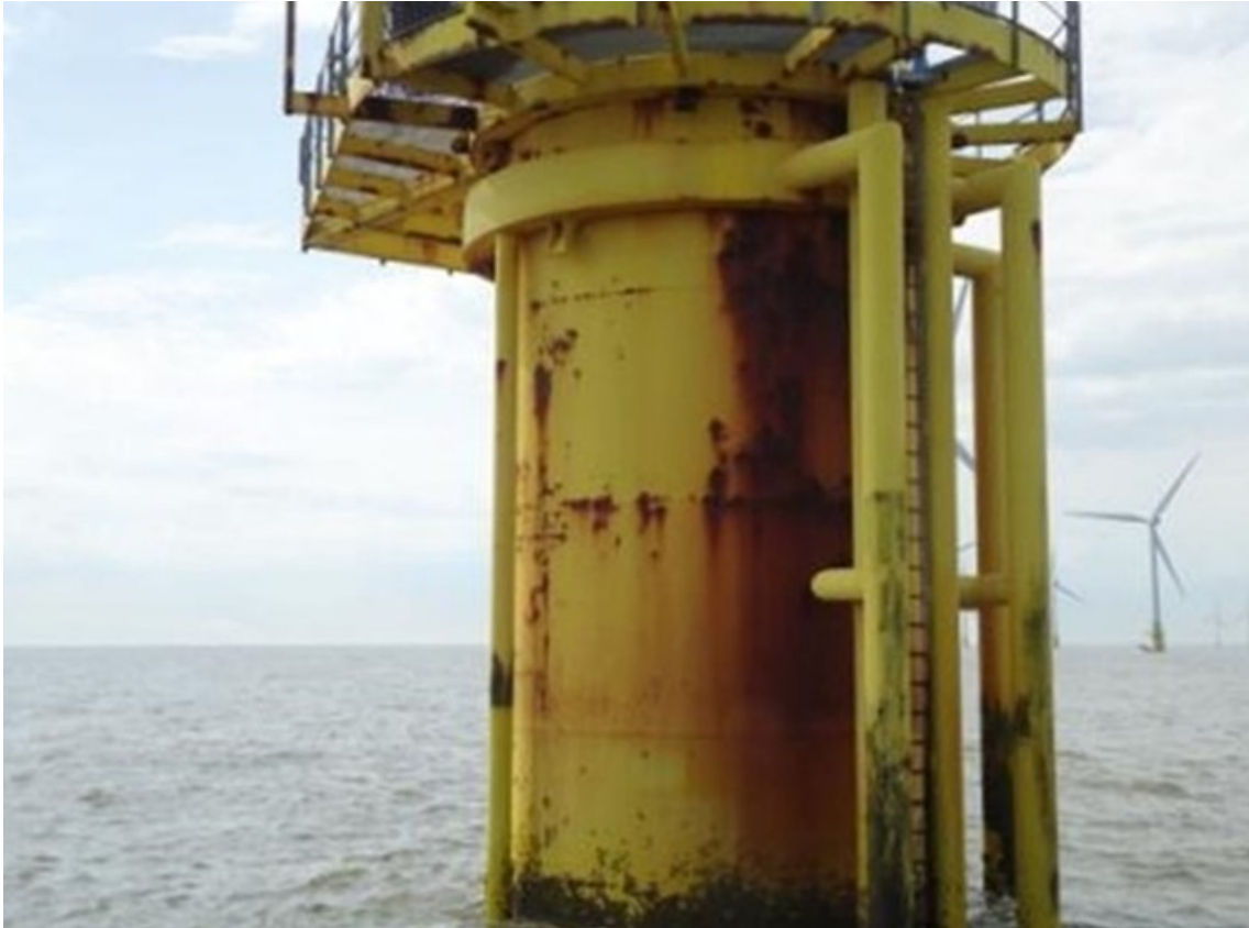
Figure 4-25 External corrosion on a transition piece at Scroby Sands wind farm (UK)
