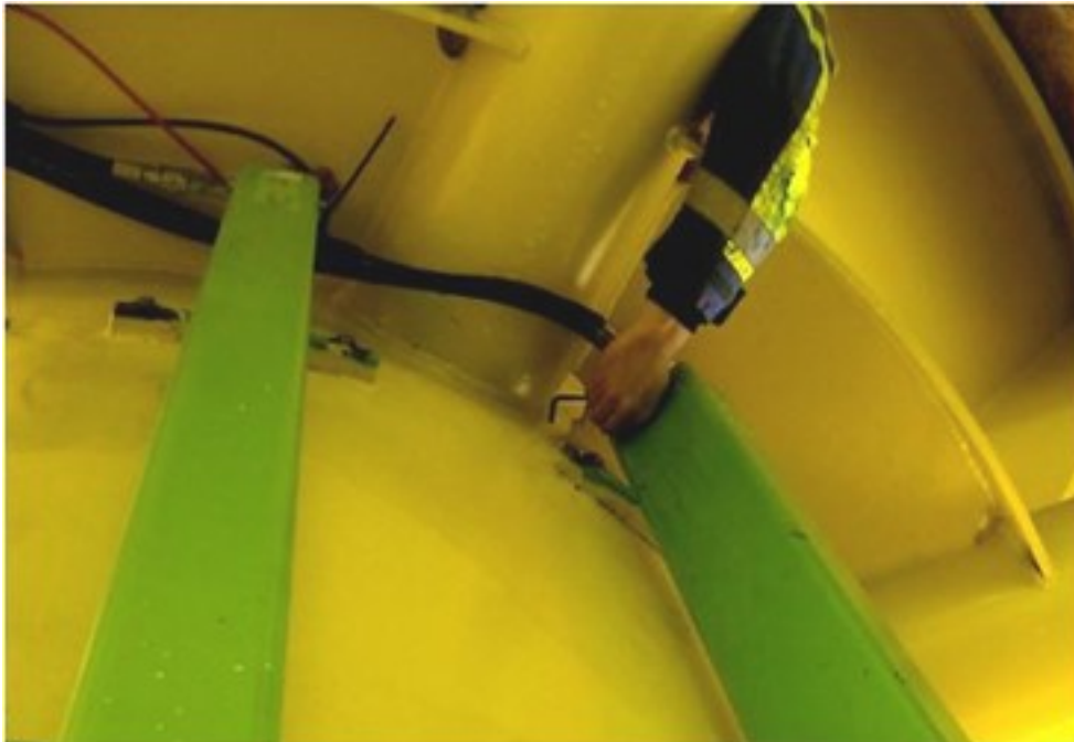
Accessibility for installation of instrument is usually better at the yard than in the field
