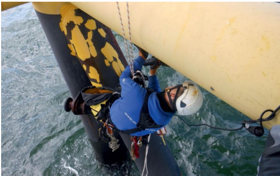
Figure 5-66 Corrosion and coating repair in the field is extremely costly and difficult
