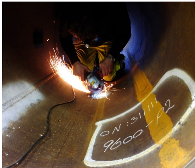
Figure 7-1 The yard can be a dangerous place especially for unprotected cables (photo: NGI)
