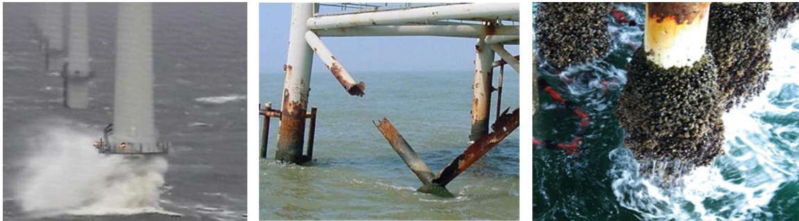
Figure 7-45 Examples of the severe conditions which can be expected at the splash zone
