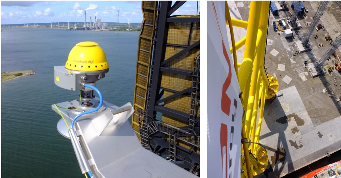
Figure 7-11 Great view when working at height installing a wave radar on TP deck (Photos: NGI)
