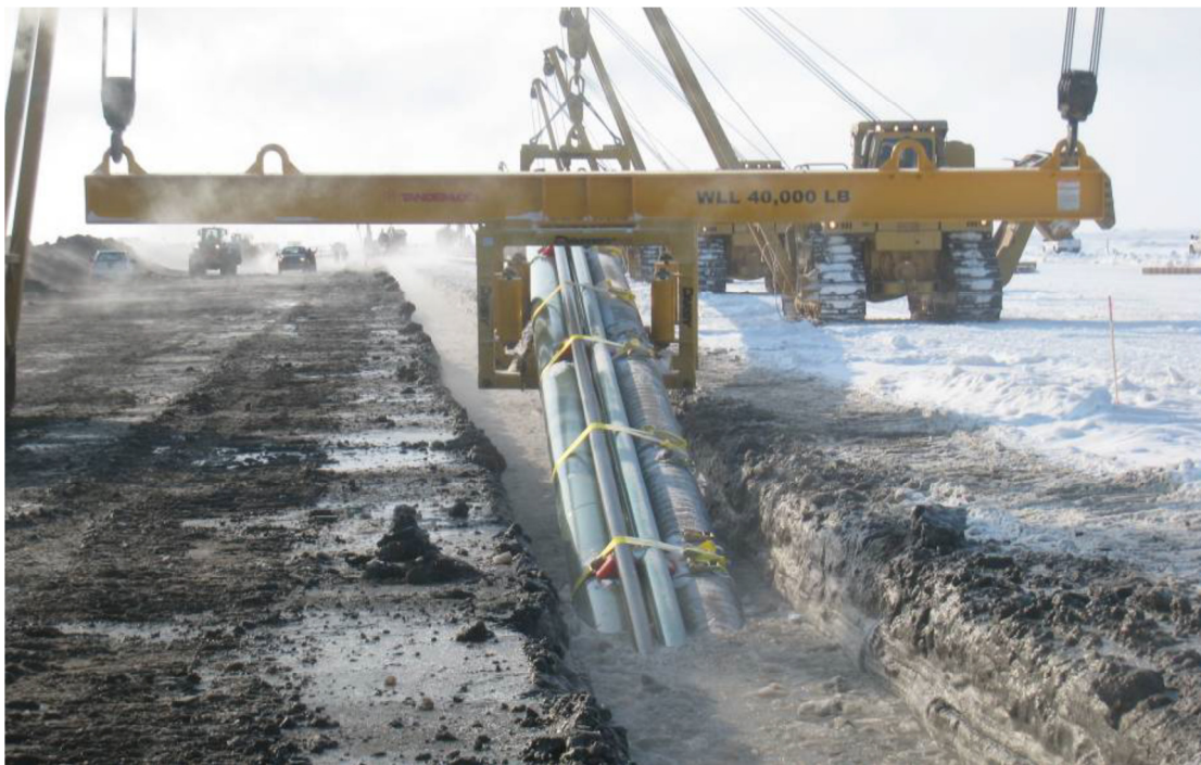
Figure 3-12: Nikaitchuq Flowline Bundle Installation [Ref. 17]
