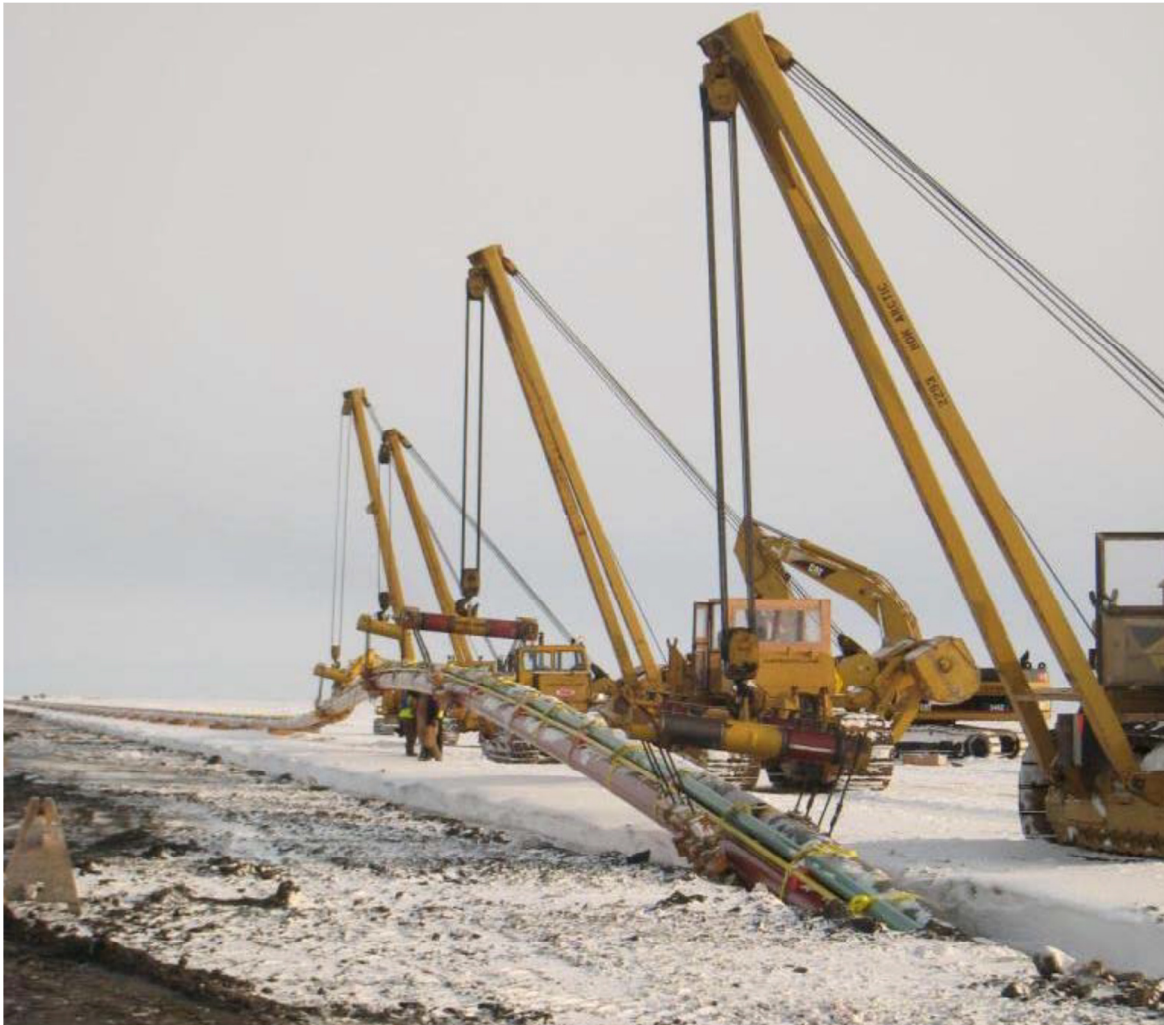
Figure 3-9: Oooguruk Flowline Bundle Being Lowered into the Trench [Ref. 16]
