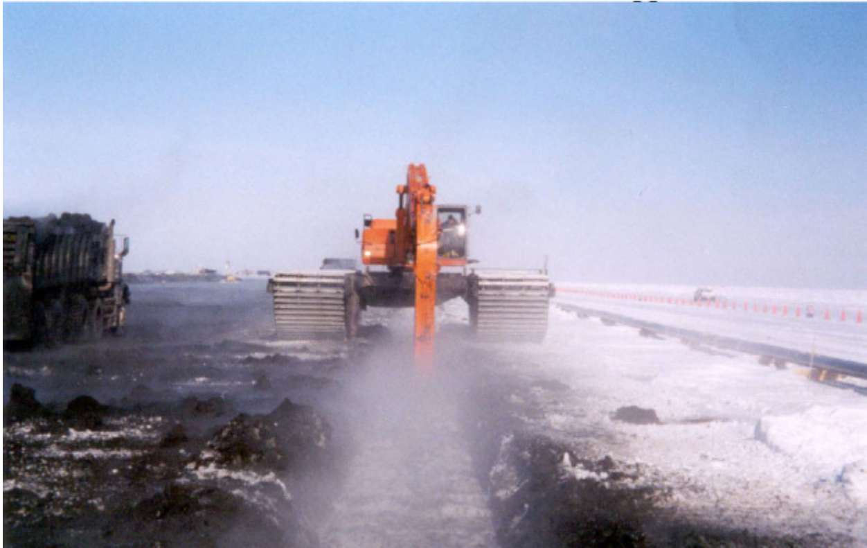
Figure 11-6: Winter excavation using Conventional Backhoe
