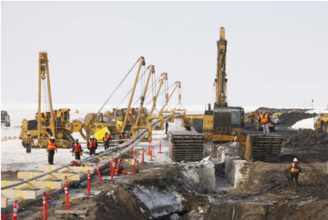
Figure 3-11: Nikaitchuq Flowline Bundle Installation [Ref. 11]
