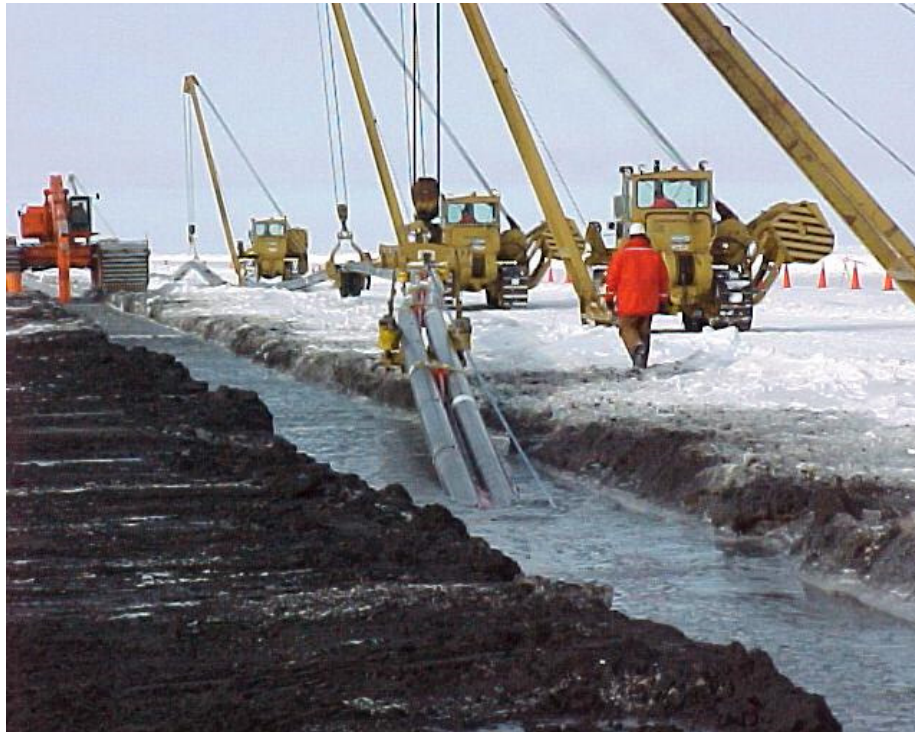
Figure 3-5: Northstar Pipeline Installation [Ref. 14]
