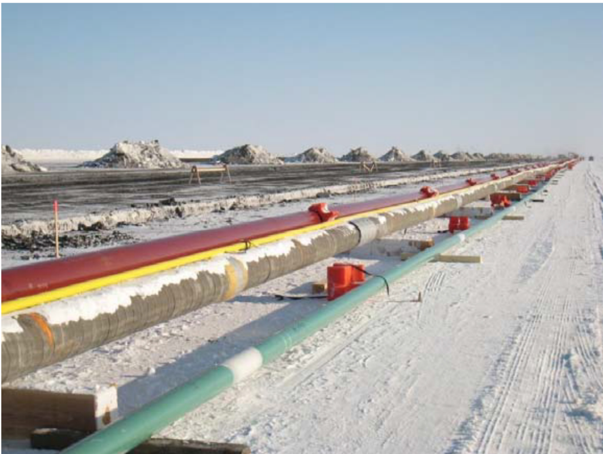
Figure 3-8: Oooguruk Flowline Bundle Fabrication [Ref. 16]
