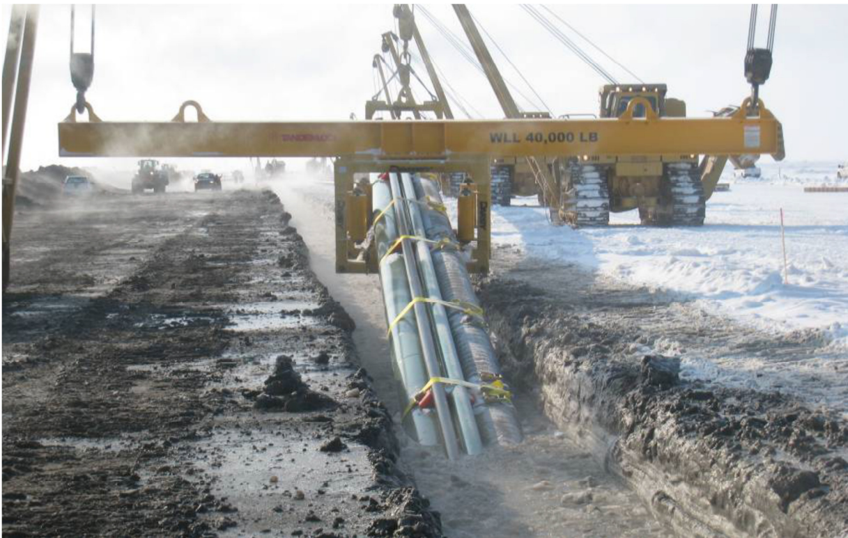
Figure 4-6: Nikaitchuq Flowline Bundle Through-Ice Installation into Trench [Ref. 17]
