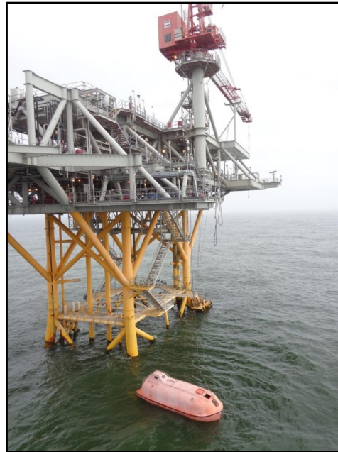
Lifeboat in the water after an inadvertent descent
