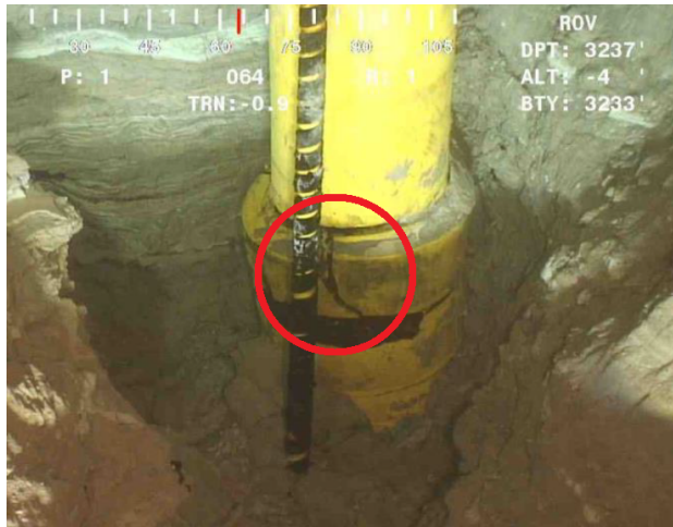
May 2016 - The load limiting joint cracked, but the leak was not identified until many hours later.
