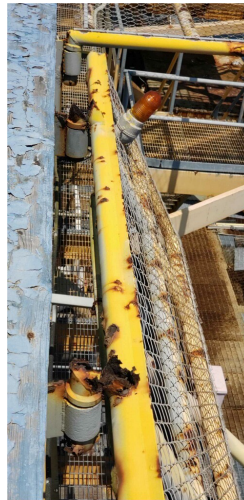
Figure 2 - Collapsed helideck skirting
