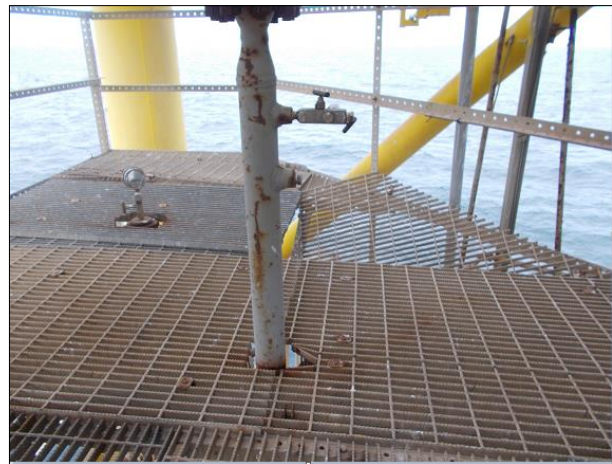
View of the loose grating from the well bay deck.
