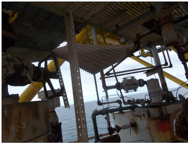
View of the loose grating from below the well bay deck.
