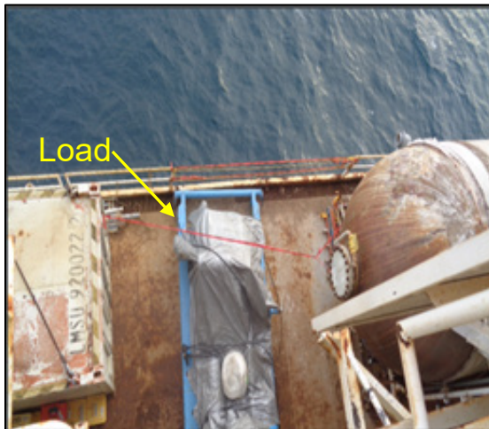
Caution tape in the center of the photograph marks the location where a handrail broke off after being struck by a 15,500 lb. load.
