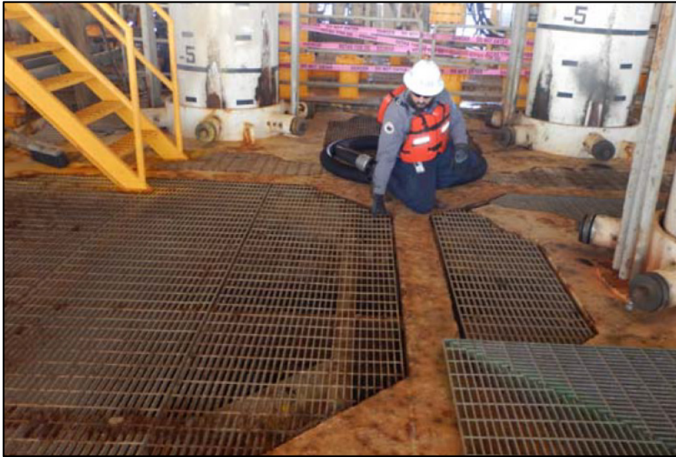
A BSEE inspector conducts a grating and open hole hazards inspection.
