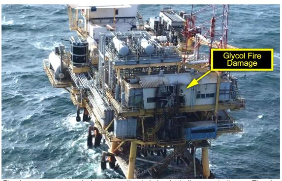
Fire damage was caused when an unattended glycol reboiler was starting up. The glycol and hydrogen condensate ignited.
