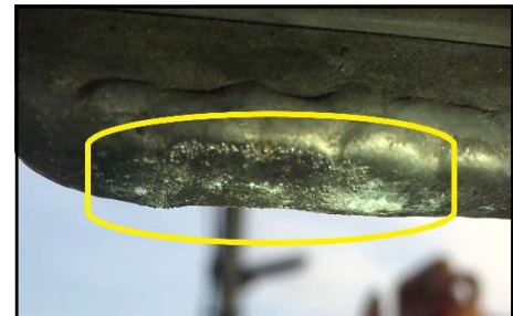
Figure 3. Lightning damage to the bottom of the skid
