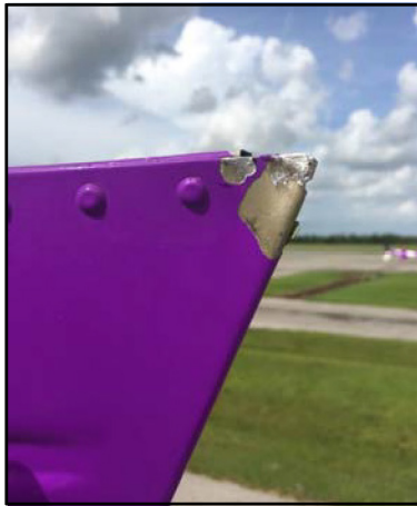
Figure 1. Lightning damage to the top of the vertical fin
