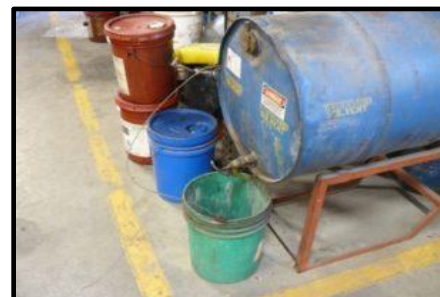
A metal container is incorrectly bonded to a plastic bucket.
