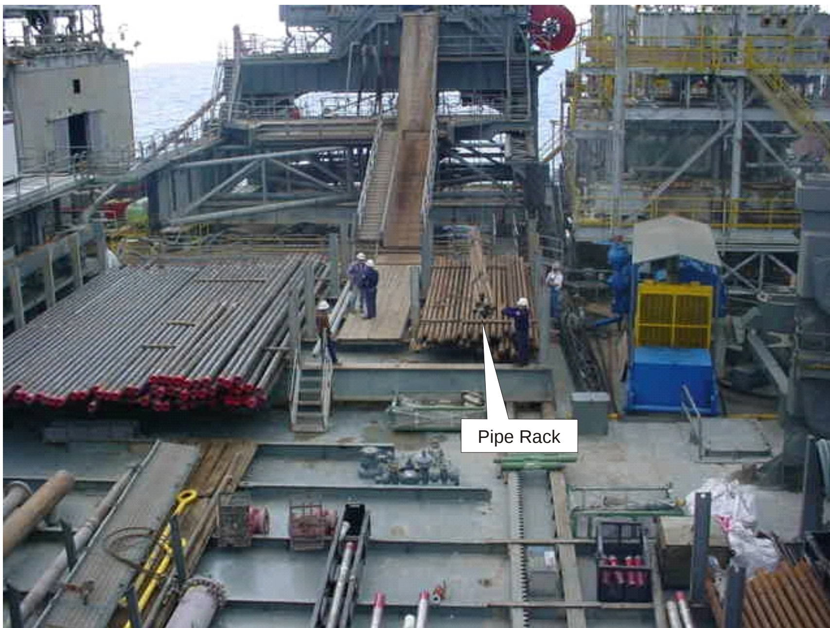
Photograph of pipe rack as seen from living quarters.
