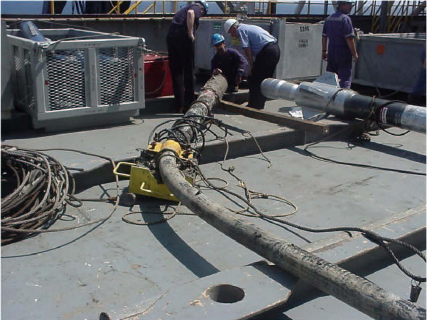
Drill pipe bending below running tool.
