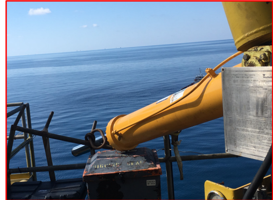
25 April cylinder failure
