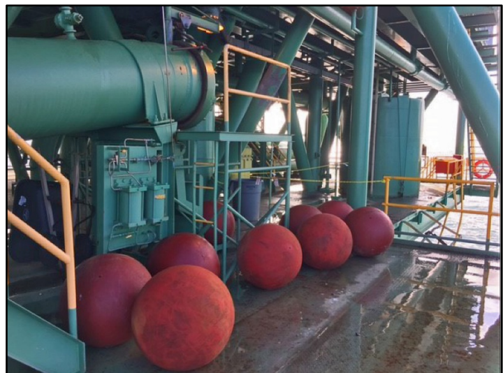
(above) Pigs located in Pig Loading Area
