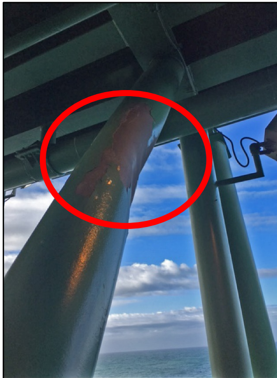
(left) Damaged/Bent Platform Structural Member
