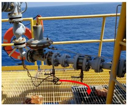
The lower left quarter of this photograph shows the twisted drain line tubing after the pressure release occurred. The red arrow indicates the pre-incident orientation of the drain line.
