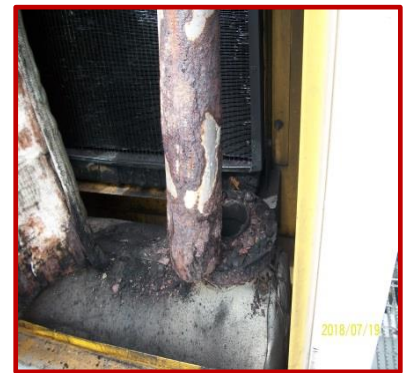
Corroded Exhaust
