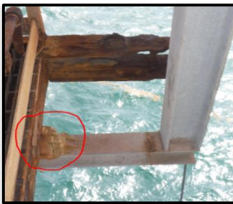
Pipe Support Connection
