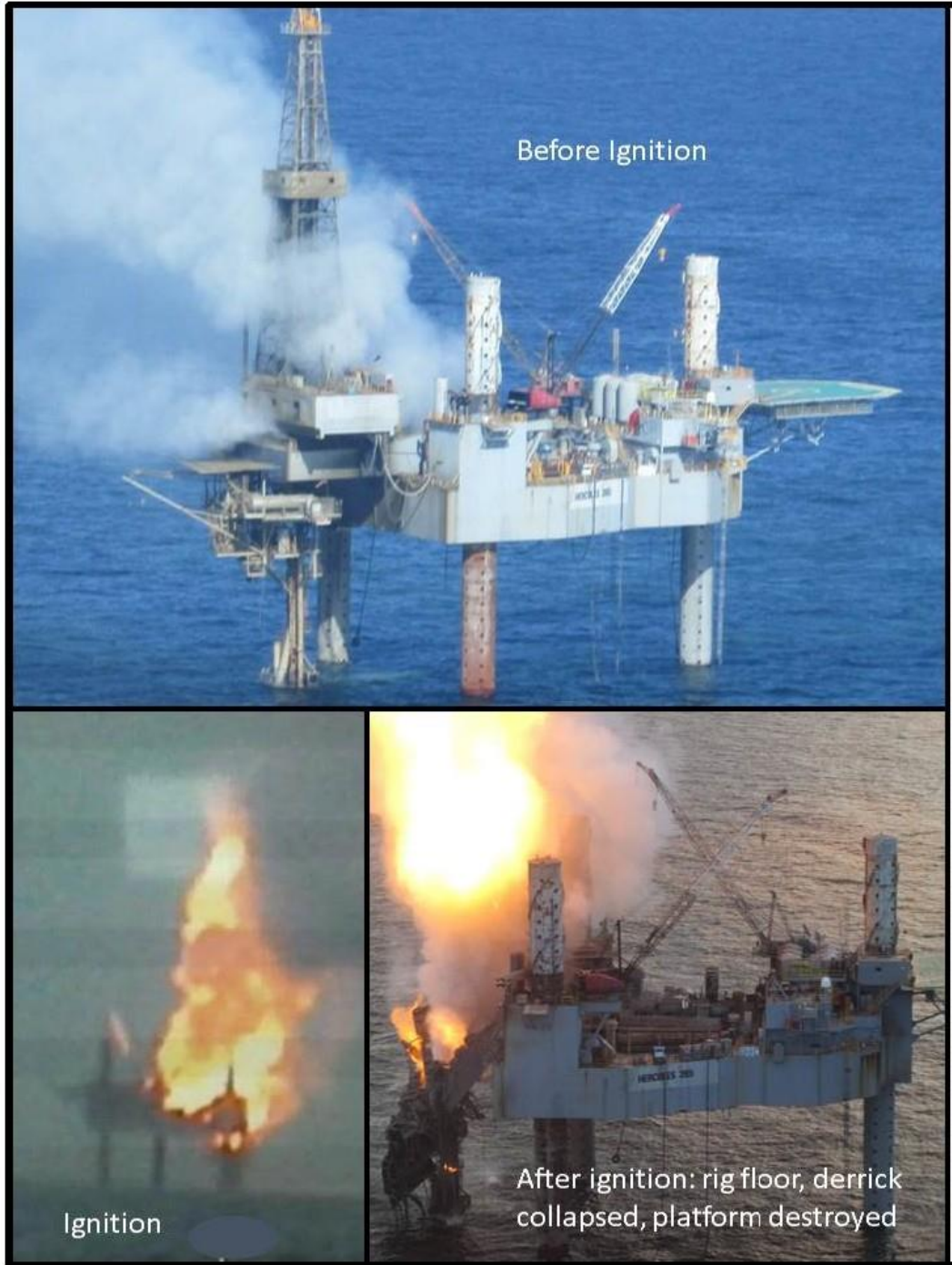
Figure 30: Rig, Platform, and Well prior to and after ignition
