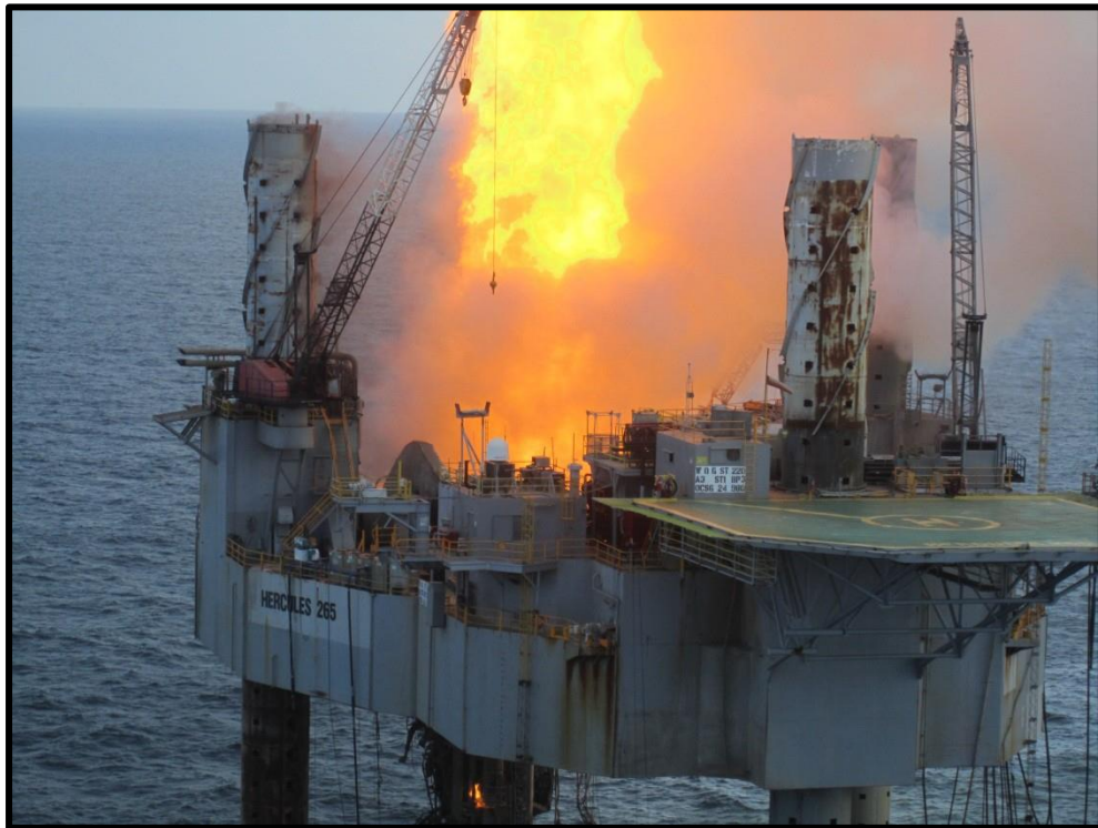
Figure 32: Blowout and fire in progress
