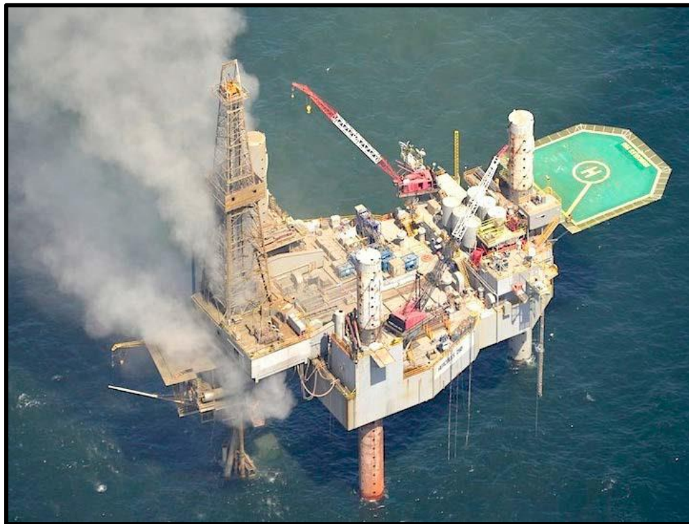
Figure 4: Hercules Rig 265 cantilevered over ST-220 “A” Platform
