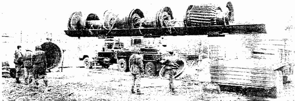
Fig. 4: Launching of the UltraScan CD into 56" gas transmission line
