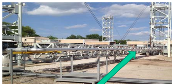
Return Line for the 2" Gas-Oil-Water Facility
