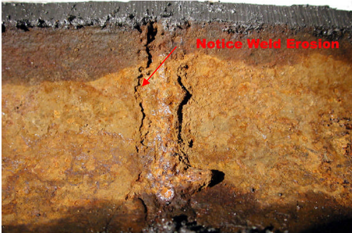
Photos #14 and #15 - Sample Photos from Line 2820
