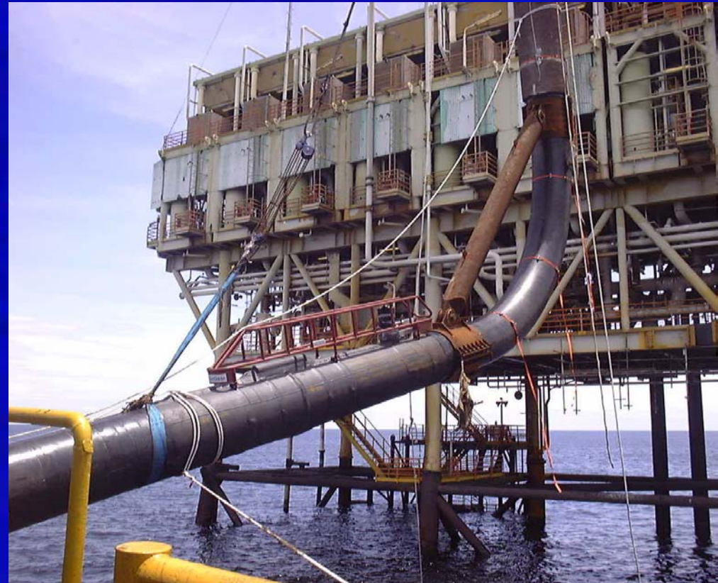
2 CorrOcean ASA, FSM (Field Signature Method) - sensors connect to outside of pipe to measure internal wall loss
