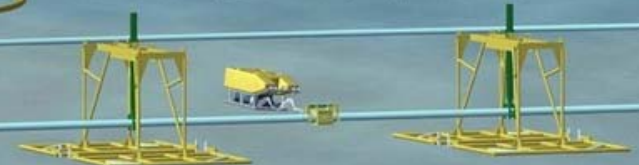
Diverless HydroClamp Pipeline Repair
