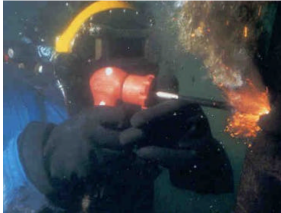
Figure 8.1: Examples of wet welding
