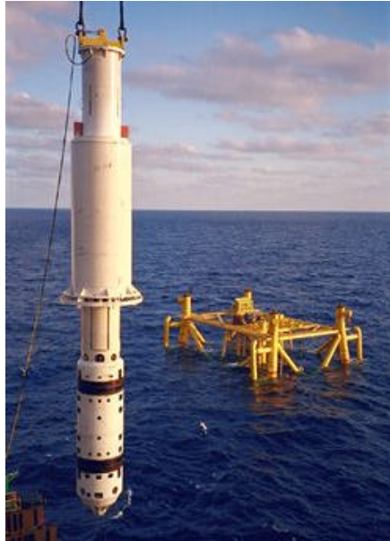
Figure 16.1: An 84-inch Oil State Hydra-Lok tool being deployed to the skirt piles of a jacket in 693 feet (211 m) of water
