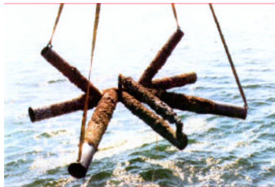
Figure 8.4: Removal of the damaged joint
