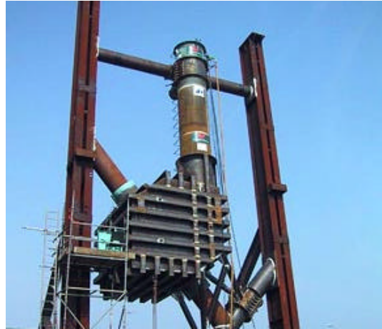
Figure 7.6: Trial fit-up of cofferdam
