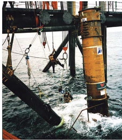
Figure 7.7: Cofferdam in position
