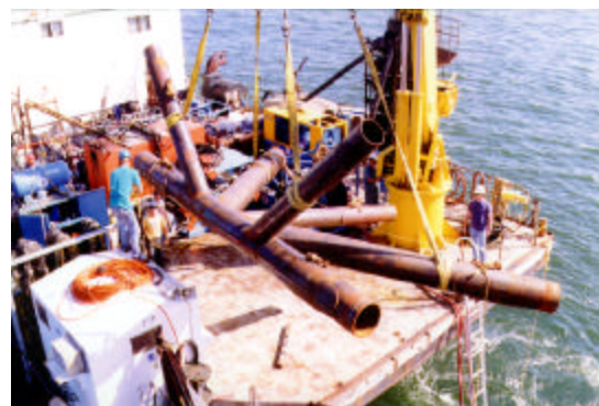
Figure 8.5: Installation of new joint
