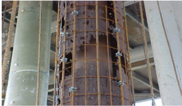
Figure 15.4: Photo of re-bar cage
