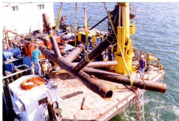
Figure 8.5: Installation of new joint
