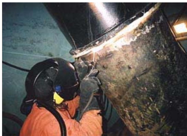
Figure 7.8: Welder at work in cofferdam
