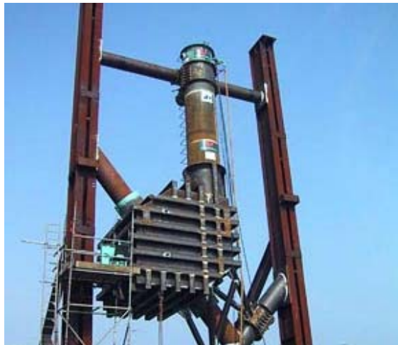
Figure 7.6: Trial fit-up of cofferdam
