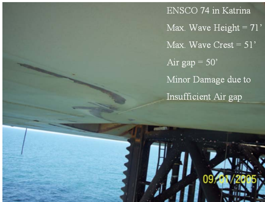
Photo 8.4.5: Bottom of Hull showing Damage from Wave hitting underside of Hull (Ref 12).
