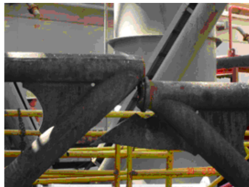
Photos: 9.17.5 Sheared Bracing.
