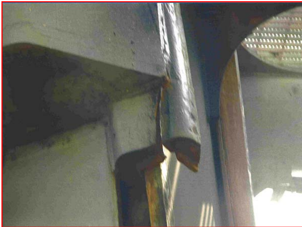
Photo 9.18.9: Lower leg guide cracked.
