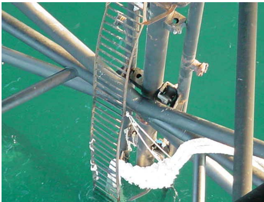
Photo 9.13.1 showing the deepwell pipe damage on the ENSCO 105.
