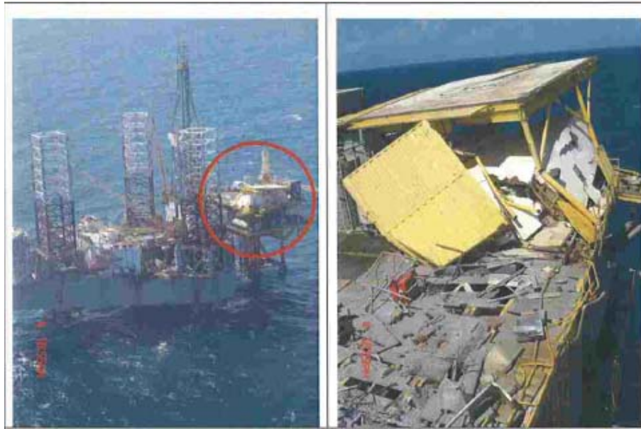
Photos 9.14.1 – Rig/Platform interface after the Hurricane Rita
