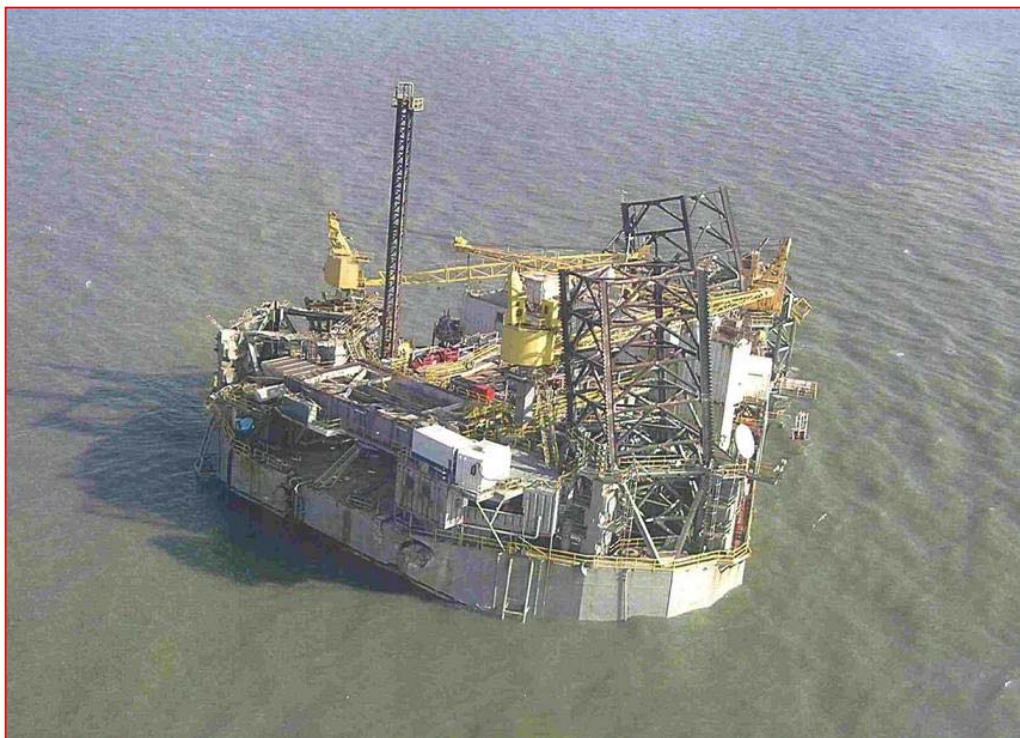
Photo 9.15.4: GSF Adriatic VII Note: Drilling package is missing and the holes in the aft end facing the reader.
