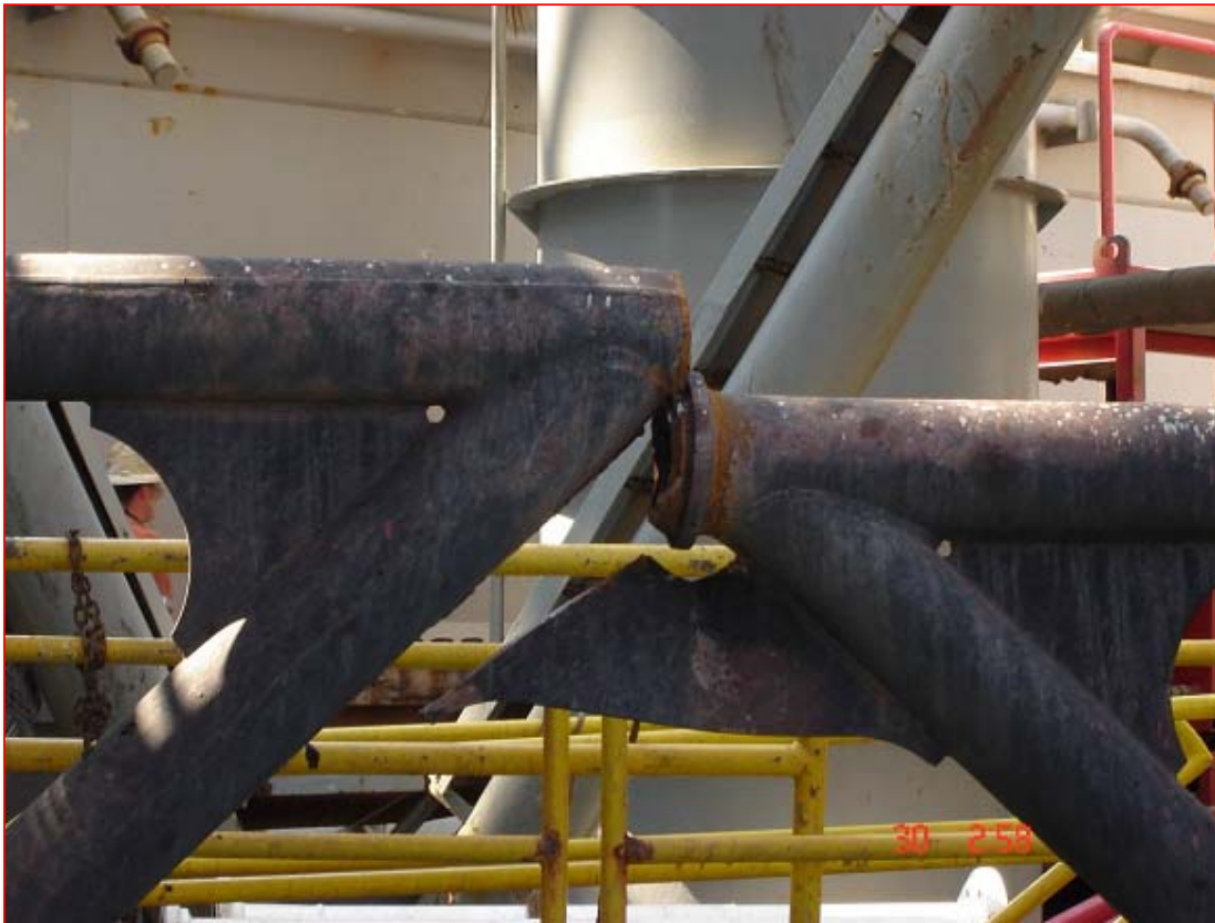
Photos 9.17.4 Some of the leg chords were bent and many of the K-braces have been overstressed. Damage was reported inside the spud cans where they interface with the legs.
