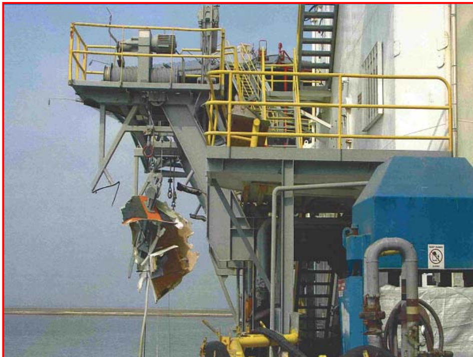
Photo 9.18.7: Lifecraft had been impacted by the storm (hanging from the davit)
