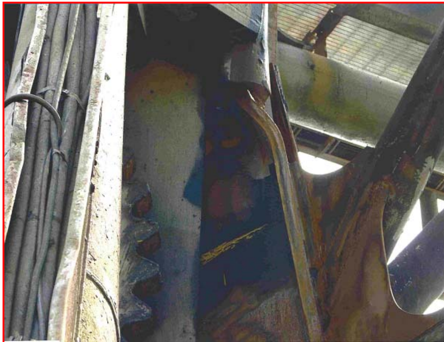
Photo 9.18.8: Damage to leg close to lower leg guide.
