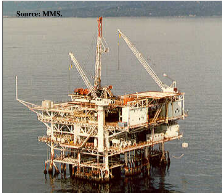
Figure E.3. Fixed Platform Structure.
