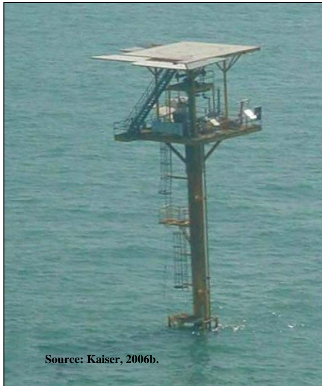
Figure E.1. Single-well Caisson Structure.
