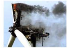
Fire caused by a short circuit. Irregular overhauling or lightning in 2004 in a Germany. Source: Der Spiegel, DPA.
