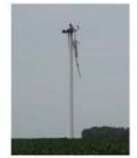
Fig. 7-5 Lightning strike damage on a wind turbine operated by Nord Energy in northern Minnesota resulted in destruction of the nacelle and the tower blades.
