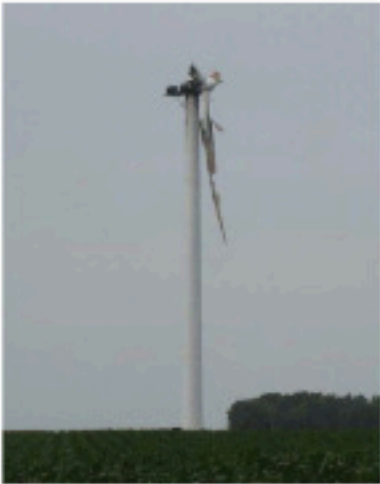
Fig. 7: Lightning strike damage on a wind turbine operated by Neel Energy in southern Minnesota resulted in destruction of the nacelle and the rotor blades.
