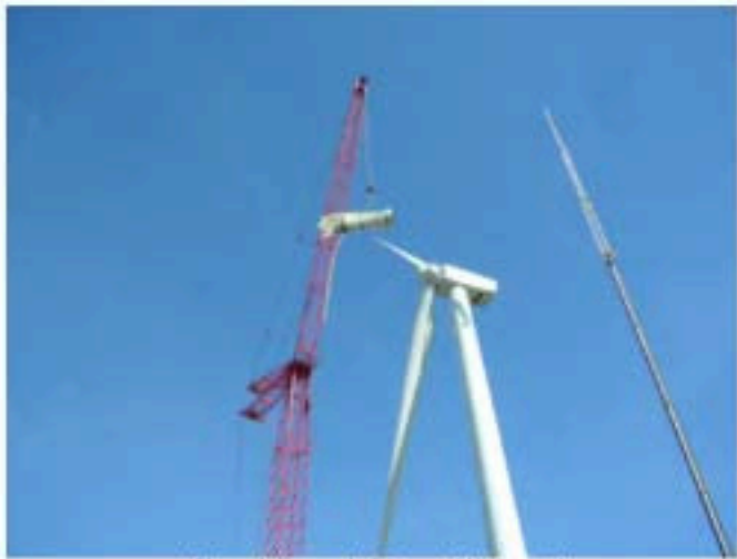
Figure 3: Removal of damaged blade root by crane
