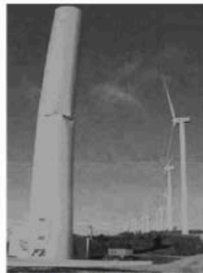
Figure 5. The loss of the turbine due to rotor bearing flaws
