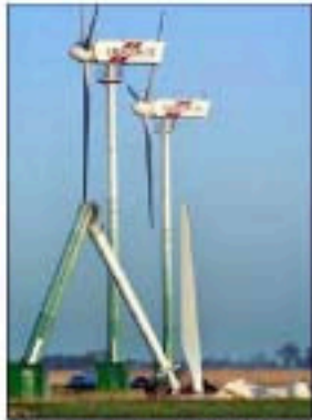
February 10, 2000: Tower Collapse Enercon E 32, 300 kW Year of construction: 1992
