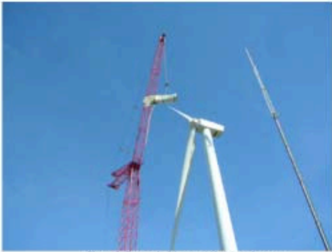
Figure 3: Removal of damaged blade root by crane
