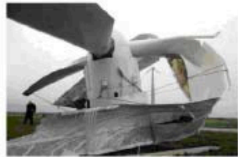
Fig. 18: Structural collapse of a wind turbine in 2002 in a storm. Source: Der Spiegel, DPA.
