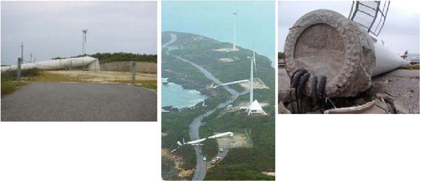
Figure 13: Failure of 7 Turbines in Japan in Typhoon Maemi (2003)
