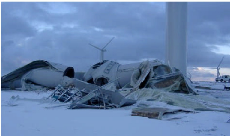
The damaged turbine. Notice the marks on the tower from one of the blades. When the nacelle crashed to the ground it was totally destroyed.
