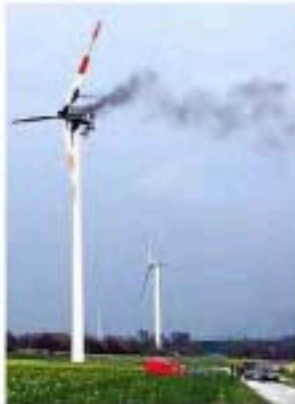
April 20, 2002: Fire VESTAS 1.5 MW Total height: 108 m Year of construction: 2000 Location: Bad Wünnenberg-Heeren near Paderborn C20020420.1.bmp
