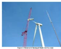
99999999.3b.bmp Figure 3. Removal of damaged blade rest by crane
