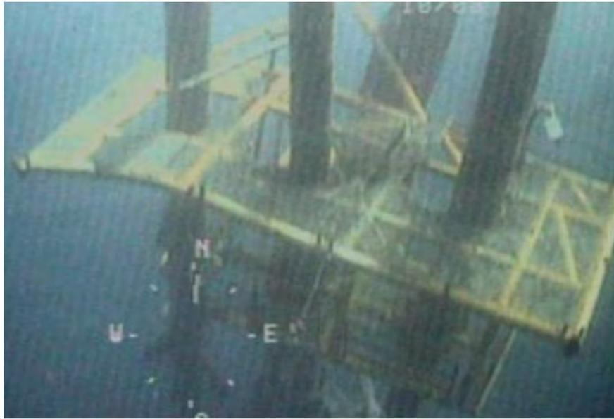
Fig. 1.1—Platform was destroyed by hurricane Ike in the East Cameron Area. (BOEMRE, 2010)
