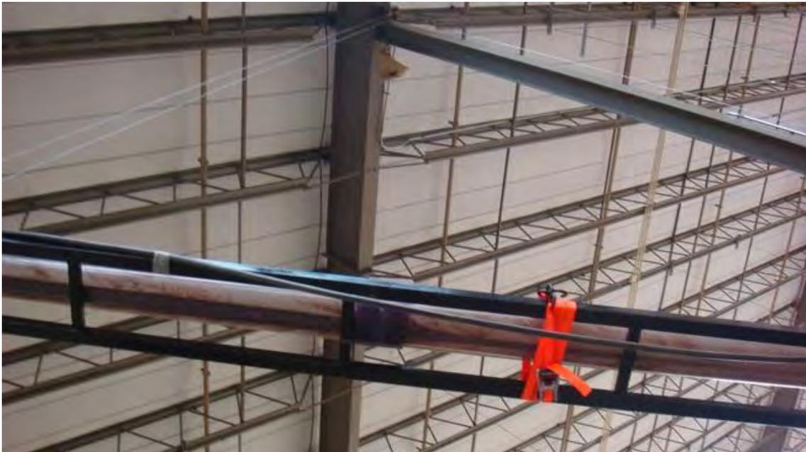
**Fig71.** Adhesion of epoxy for a slant pipe at middle section.
