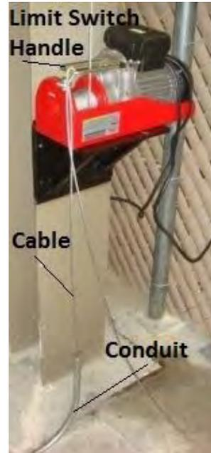
**Fig48.** Limit switch mechanism at hoist.
