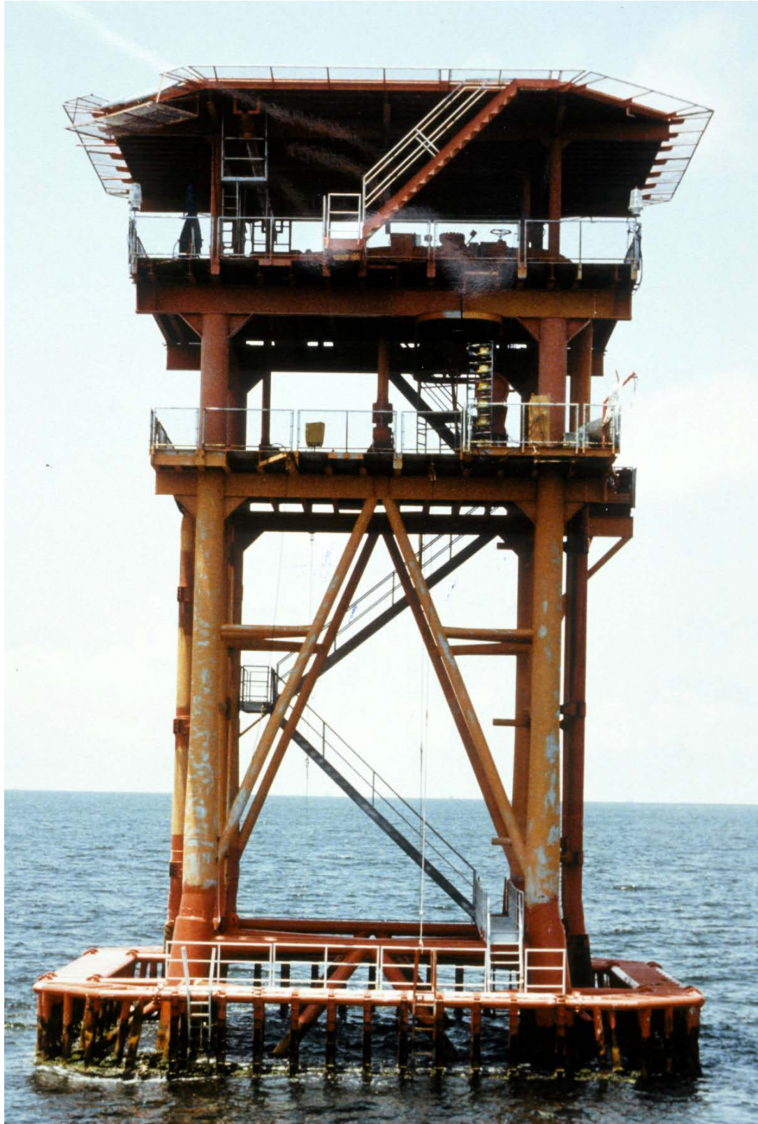
South Timbalier 52, The T-23 Platform
