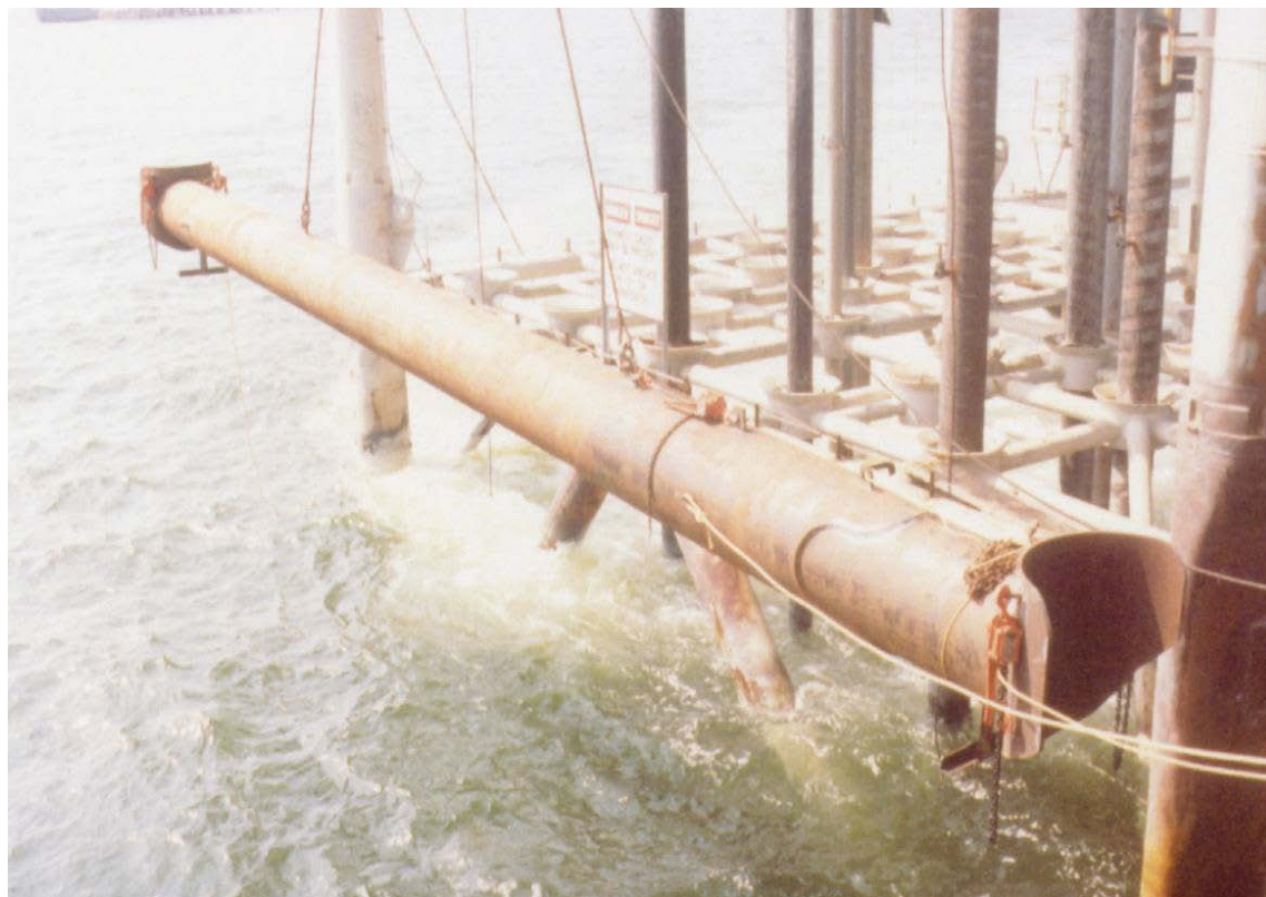
Samaan A Structure, Offshore Trinidad, -125' Elevation Telescoping Horizontal Assembly
