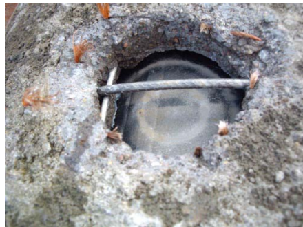
Figure 13 – Local weight coating removal on a pipeline with an HP water jet tool
