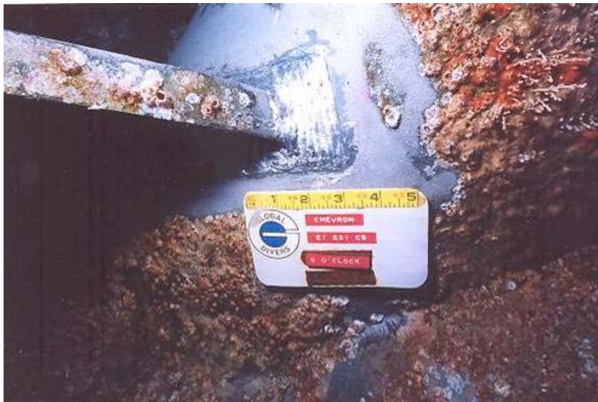
Eugene Island 231 CB, Completed Repair
