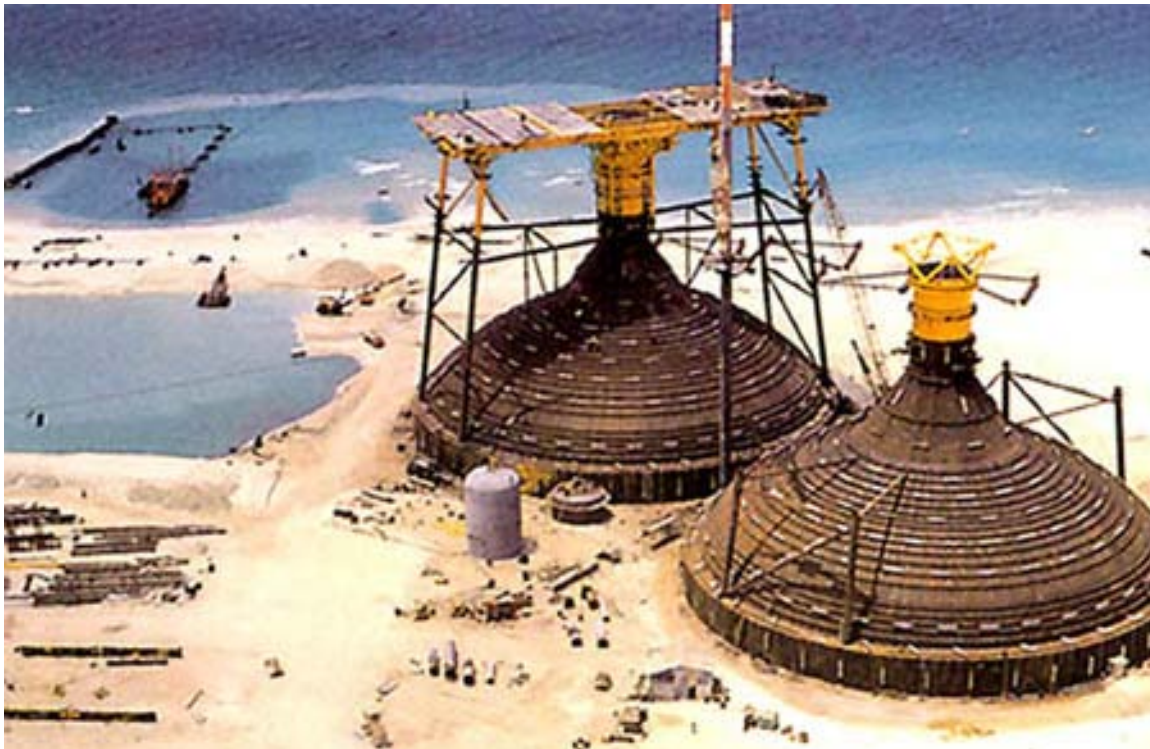
Khazzan 2 and 3 under construction at Chicago Beach, Abu Dhabi
