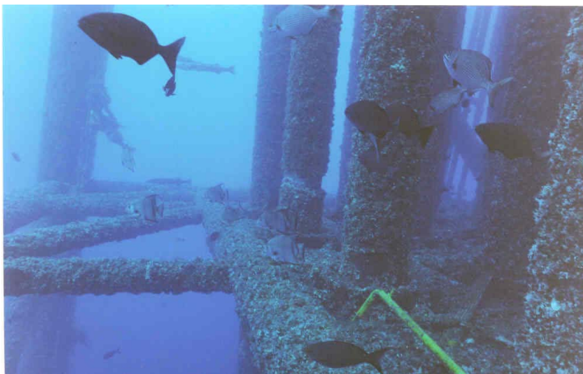
Ship Shoal 291 A, Conductor Bays Filled with Conductors
