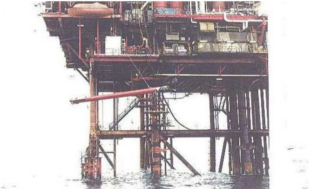
Montrose Structure, North Sea, New 30" Brace Being Lowered to the Water
