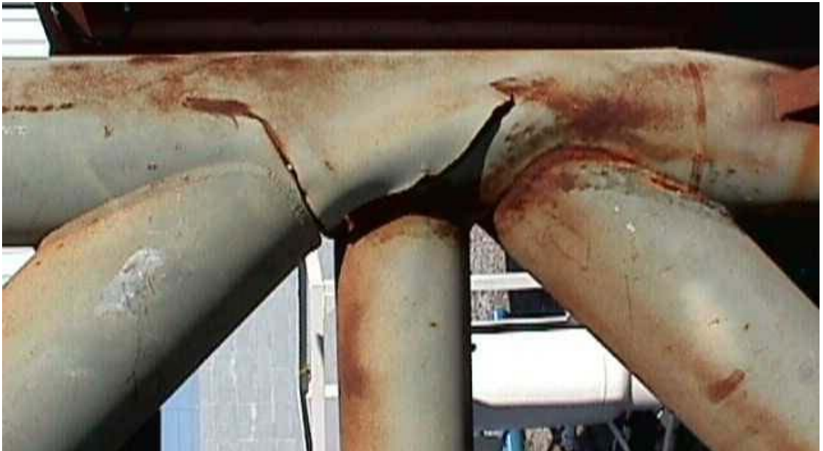
South Timbalier 52, Type T/K node removed and cleaned up
