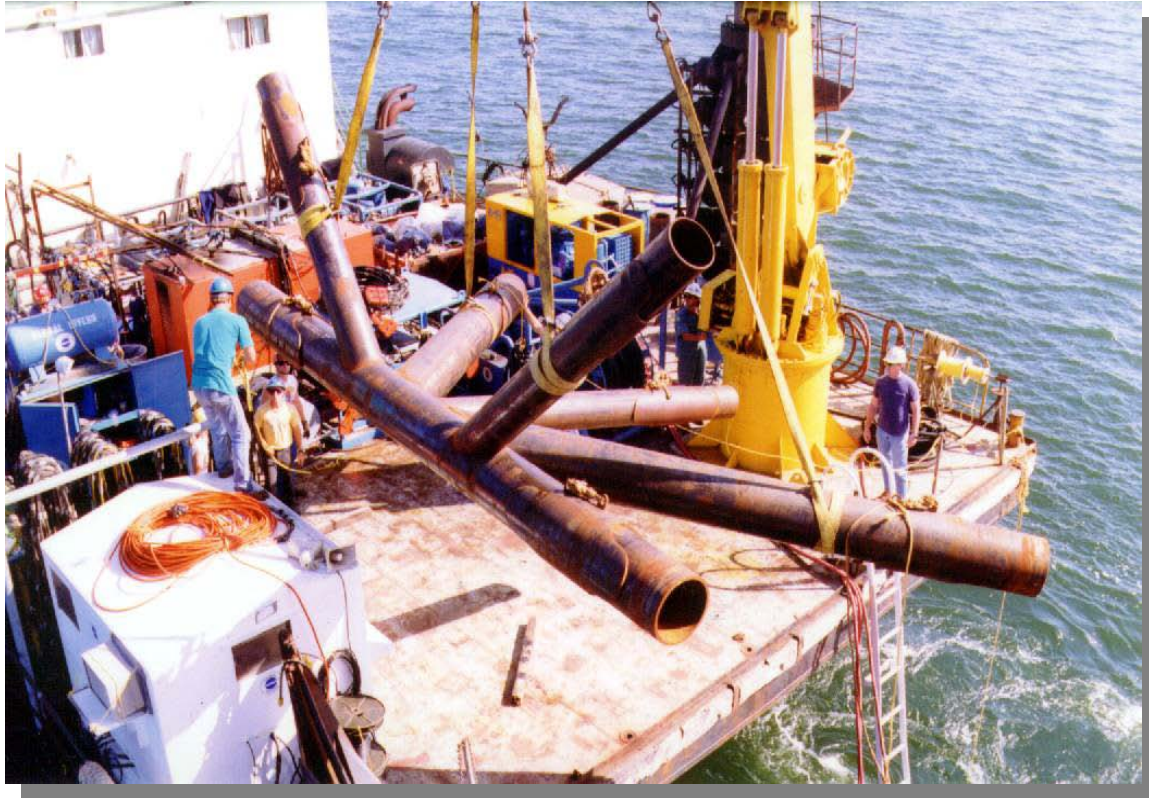
South Timbalier 52, Redesigned T/K Node Ready to be Launched
