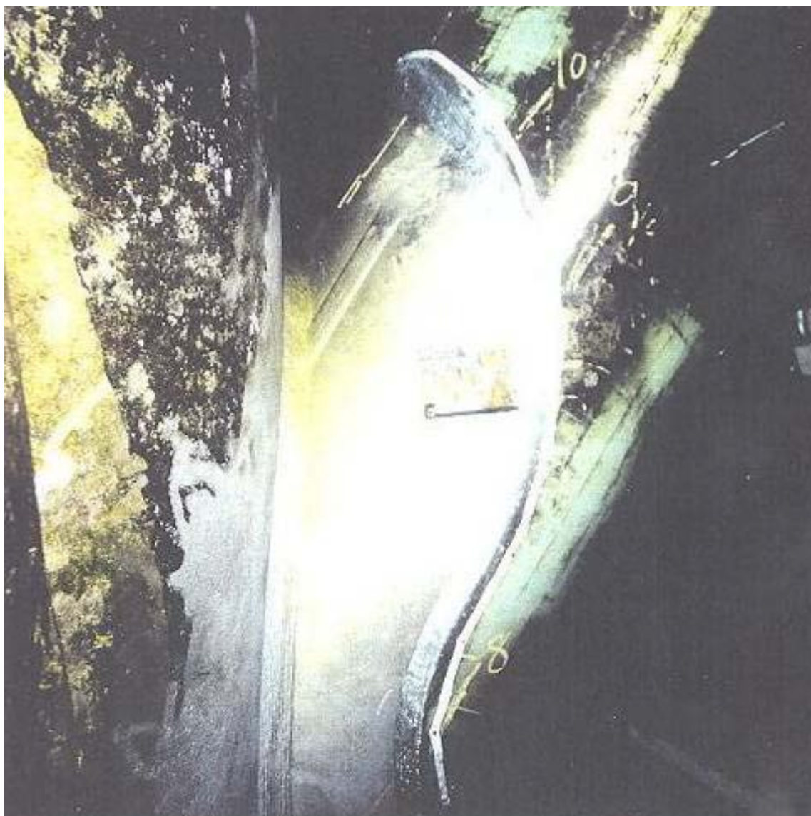
Montrose Structure, North Sea, Single Lobe Scallop Sleeve Used to Accommodate Shore Stub Length and Minimize Overhead Welding
