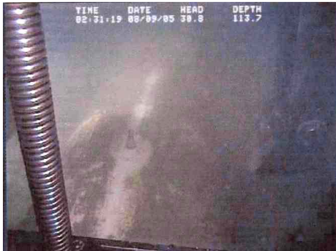
Figure 12 – A stud weld done by an ROV through the epoxy coating on a live subsea pipeline
