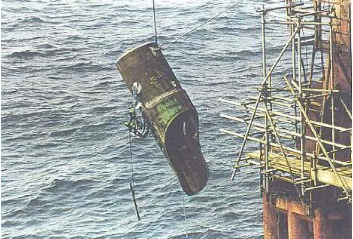
Montrose Structure, North Sea, Scallop Sleeve Going Down for Trial Fit on Stub
