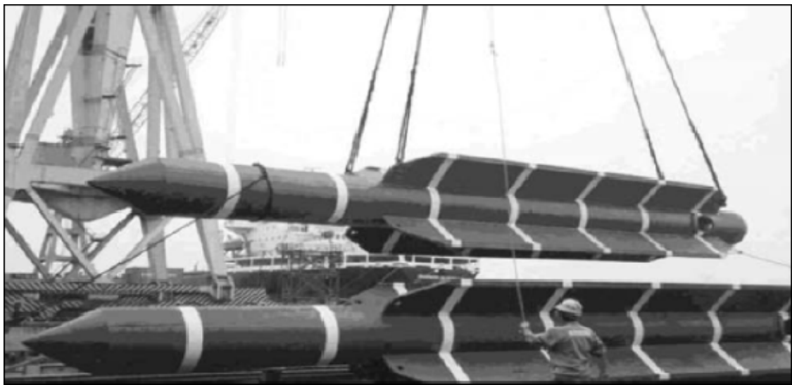
Figure 5.1: Typical Torpedo Pile Geometries as used by Petrobras in the Campos Basin
