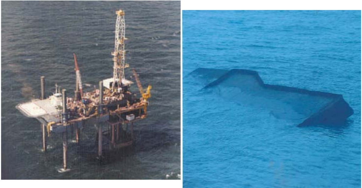
Figure II.3: Nabors Dolphin 105 Pre and Post Hurricane Lili Event
