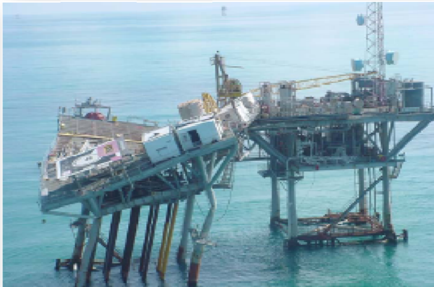
Figure III.6: Damage to an offshore structure during extreme event
