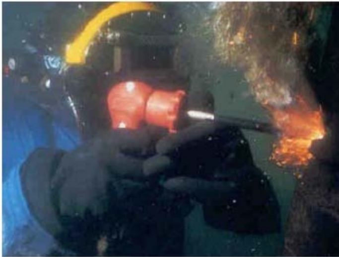
Figure VI.4: Example of wet welding repair
