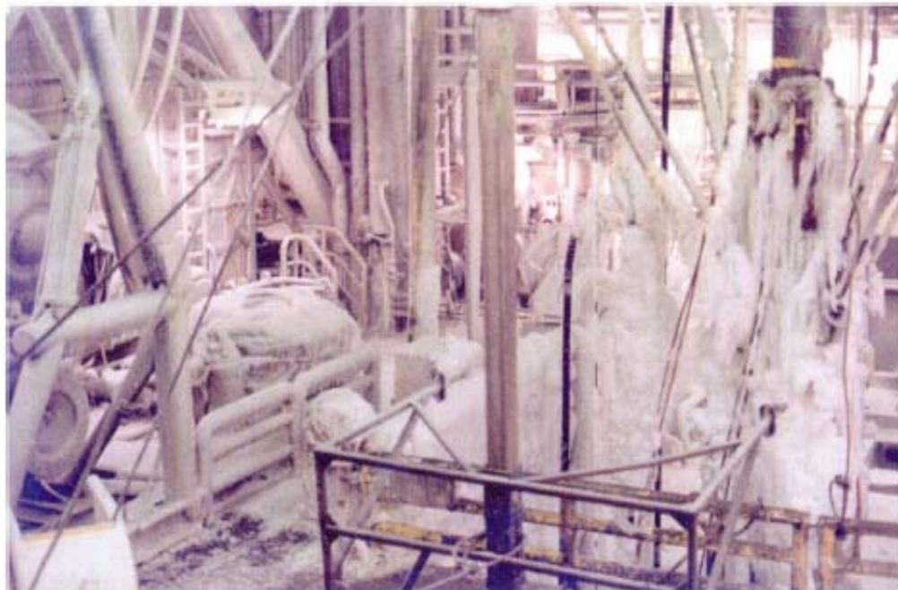
Figure X.1: Sea spray icing on the Ocean Bounty (1979-1980 Winter)
