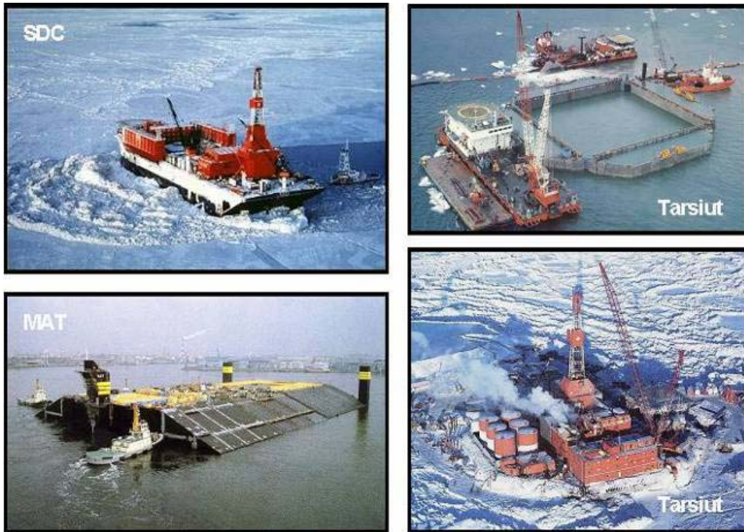
Figure X.5: Arctic Caisson Drilling Structures
