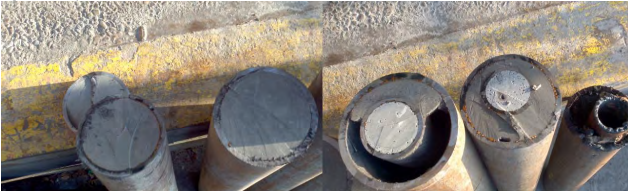
Figure 25: Pipe #3, 20 foot Perm Test
