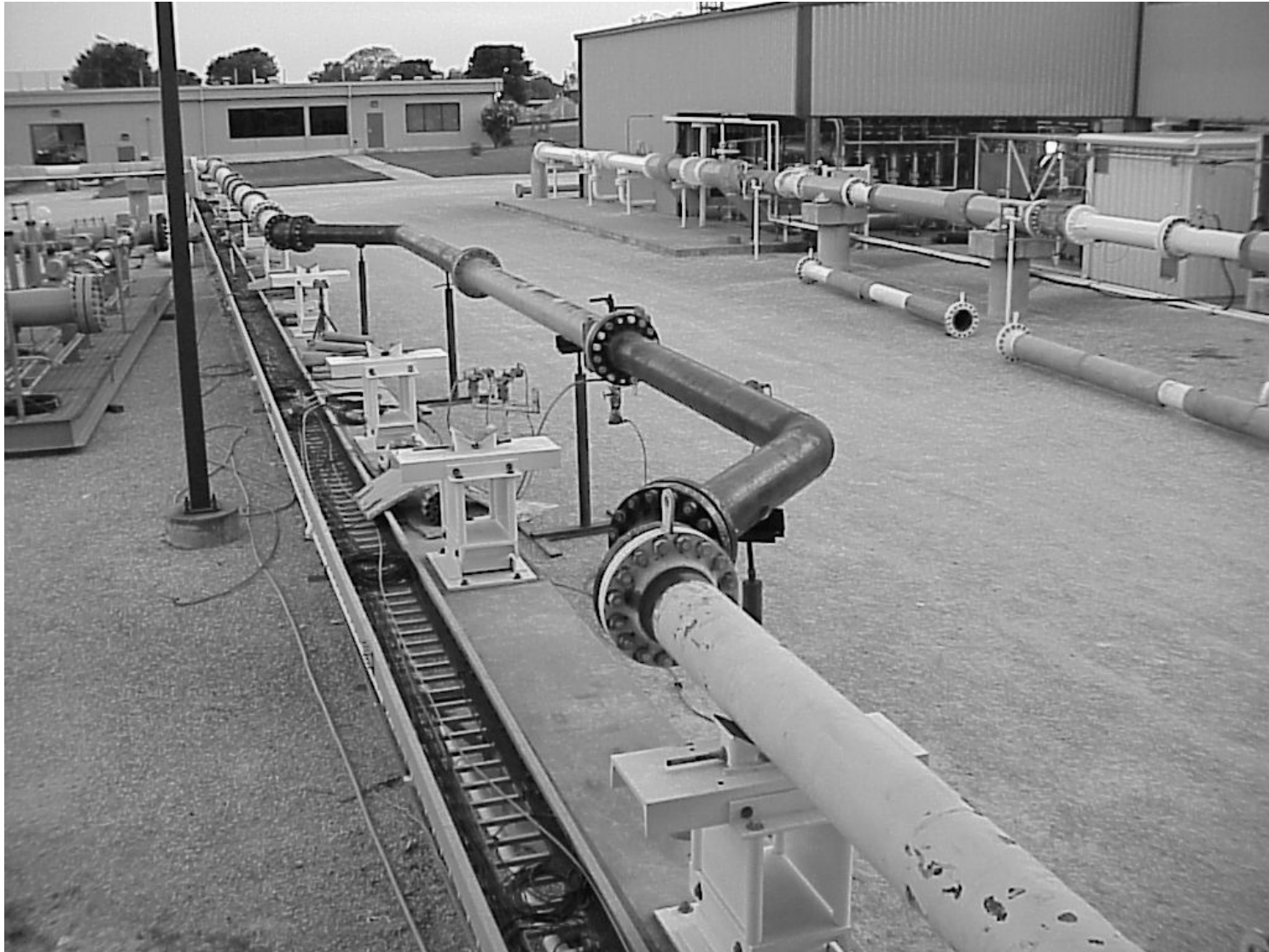
MRF HPL Test Installation
