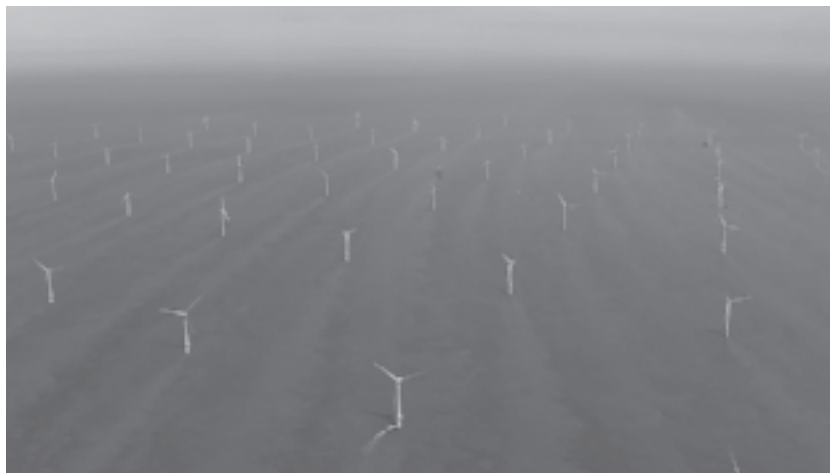
FIGURE 2-7 300-MW Thanet wind project off the southeast coast of England. (SOURCE: Vattenfall; photograph by Lavernder Blue.)
