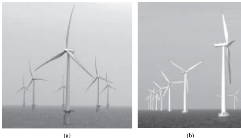
FIGURE 2-3 Common offshore wind turbines: (a) Vestas 3-MW turbines with 90-m rotor diameters and 70-m hub heights at Thanet in the United Kingdom. The turbines are on monopile foundations. (b) Siemens 2.3-MW turbines with 83-m rotor diameters and 69-m hub heights at Nysted off of Denmark. These turbines are on gravity-base foundations. (SOURCE: Vestas, Siemens.)
