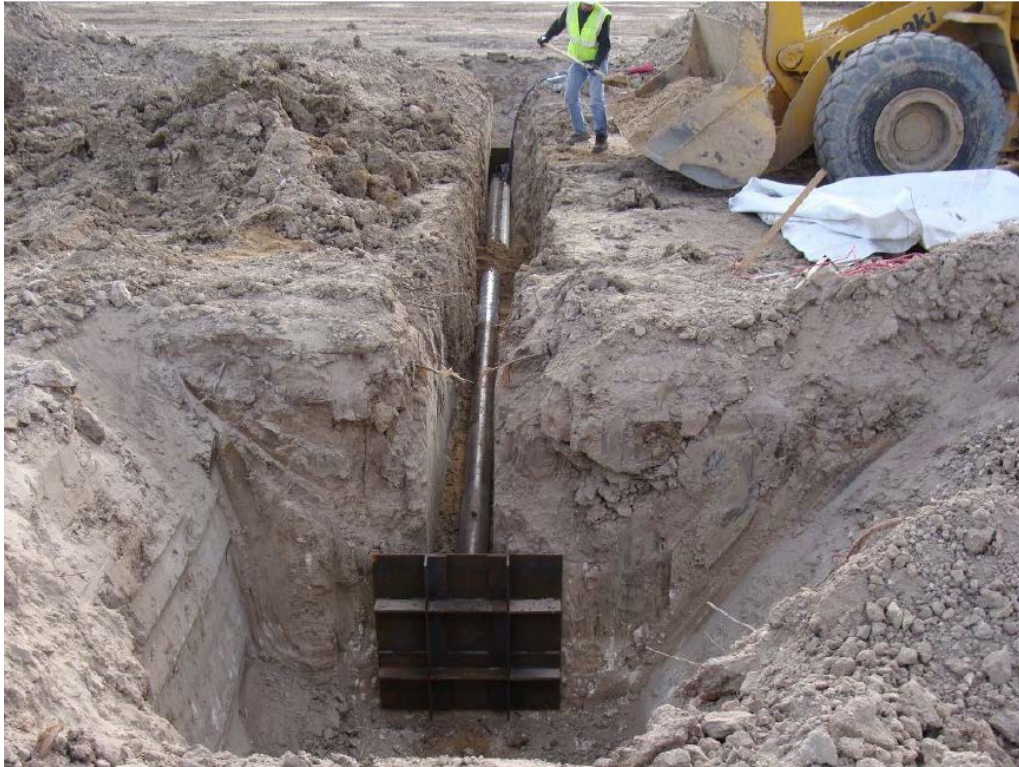
Figure 6.13: View of the Pipe (Sancio et al., 2011 [117])
