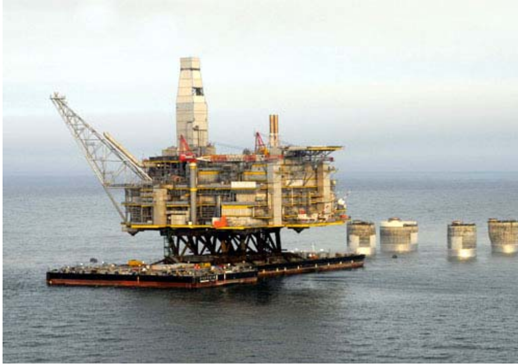
Figure 3-6: Installation of PA-B Platform, Sakhalin 2 (JSC Gazprom, 2007a)
