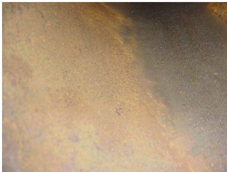
Line 25 – Internal Pipe Photos
