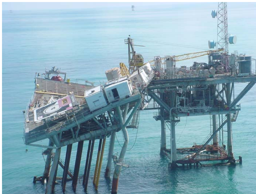
Figure 6 – Fixed Platform Damaged by Hurricane Lili
