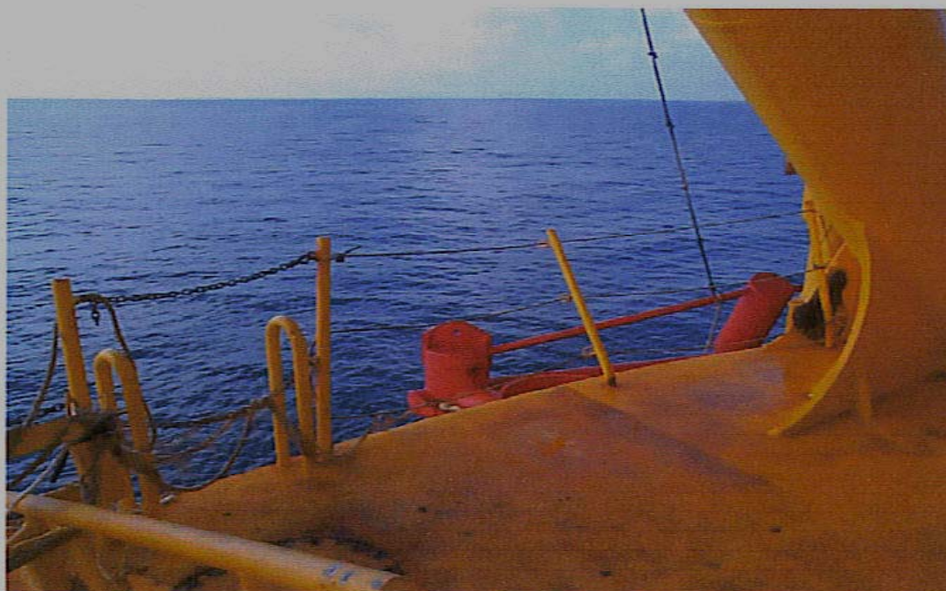
Picture 2.6-3 – Missing or Bent Handrails due to Hurricane Lili
