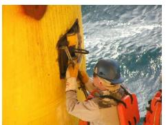
66" x 2.25" leg can 12" x 12" hole cut out stabbing guide
