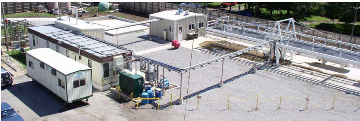
Figure 4.1: Overall view of hydrate facilities
