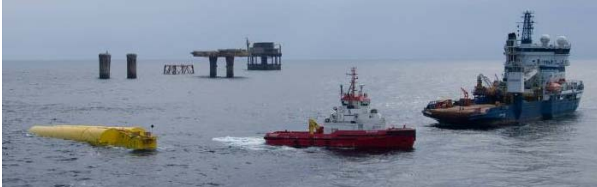
Figure 2.5: Towing Buoyancy Tank Assembly to site (Ref: Aker Solutions, Stavanger & Stord 2008)
