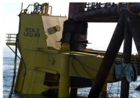
BTA locked in position on to DP2 jacket
