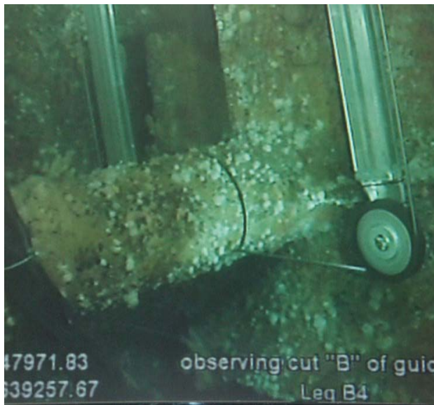
Figure 2.3 ROV Diamond Wire Tool
