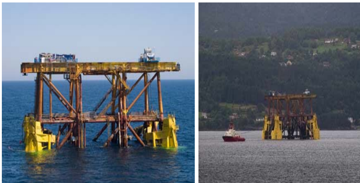
Figure 2.17 Frigg DP2 Platform Removal
