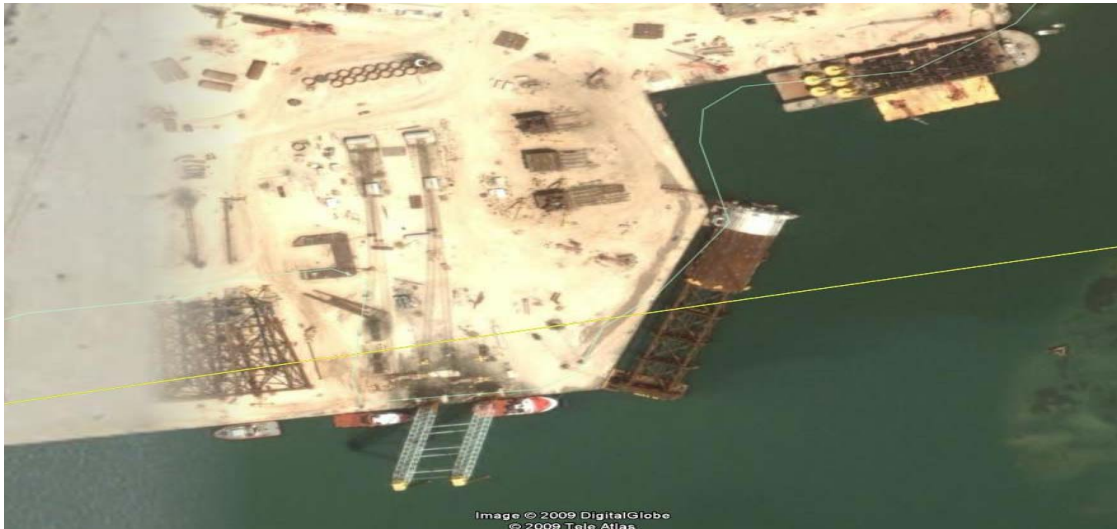
Figure 3.3 Gulf Marine Fabricators Yard (Photo courtesy of Gulf Marine)
