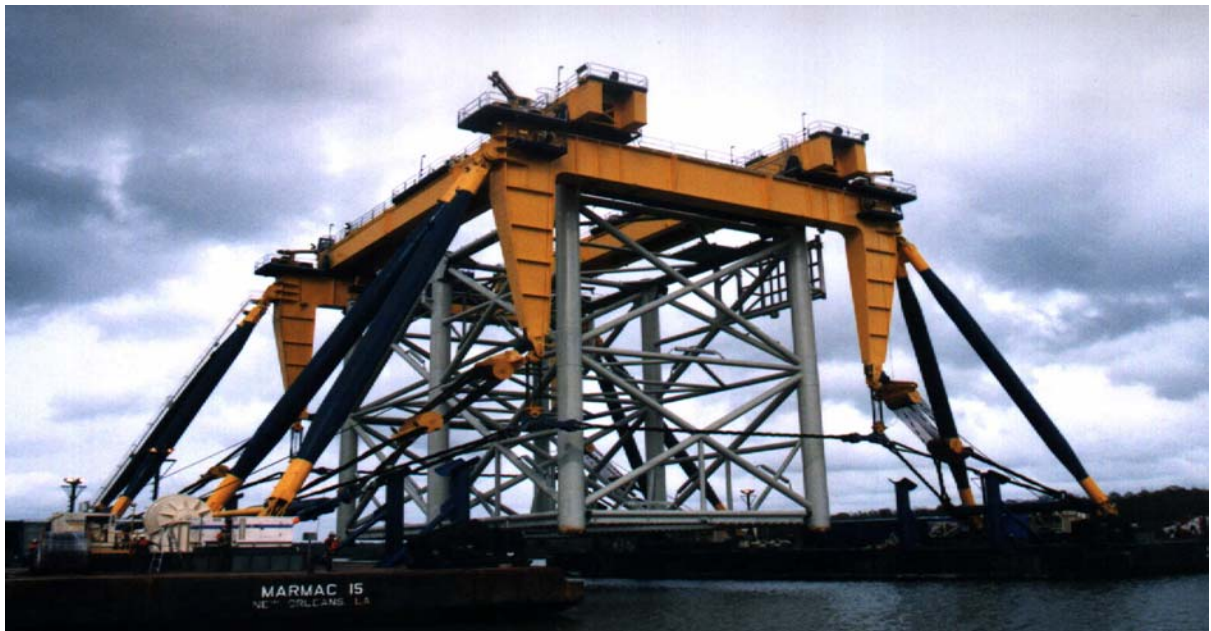
Figure 2.13- Versatruss Jacket Lifting System
