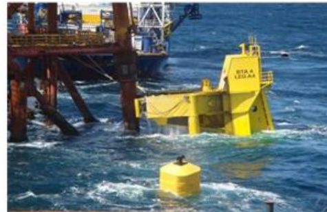
BTA upper guide contacting the DP2 jacket
