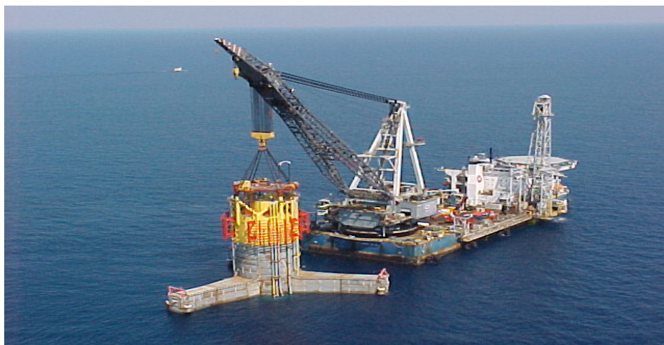
Figure 3.23 TLP Installation
