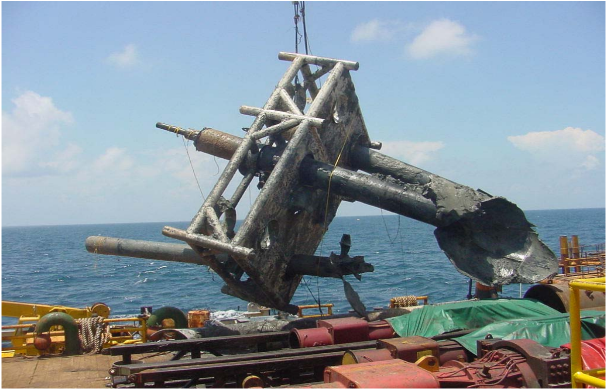
Figure 2.1 Template removal – Explosives (Photo courtesy of Demex International)
