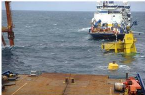
BTA was pulled slowly towards the DP2 jacket
