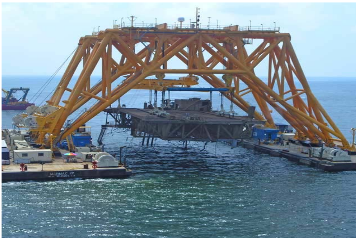
Figure 2.14- Versabar VB 4000 Bottom Feeder Lifting System (Photo courtesy of Versabar)
